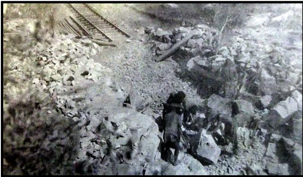
Fig. 4.4. Construction of the Selati Line north of the Sabie Bridge in 1911 (Stevenson-Hamilton Collection, Skukuza Archive in Pienaar, 1990).
