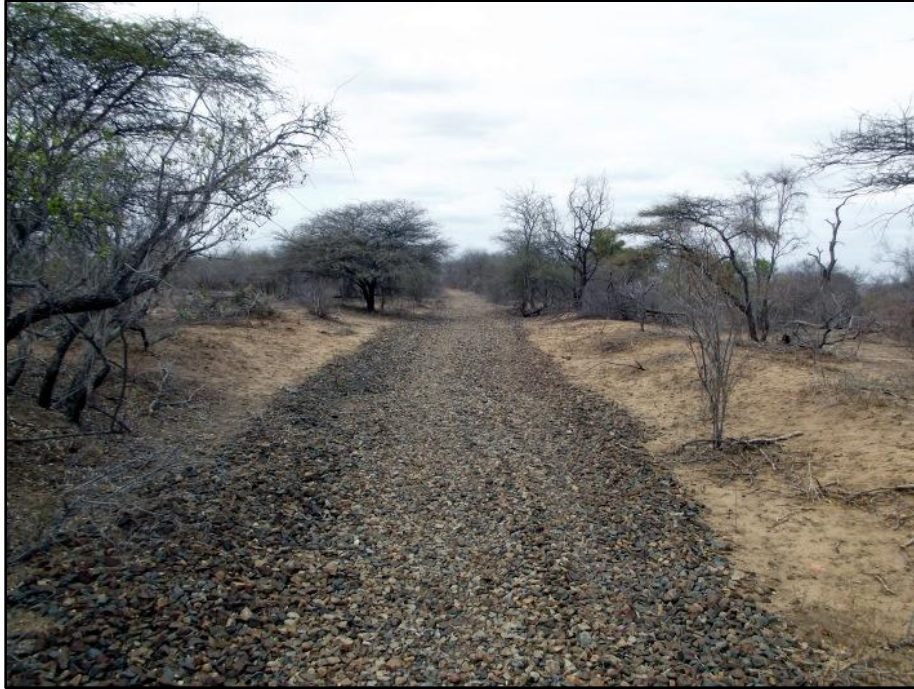
Fig. 7. Site KSS 4. The historic Selati Railway Line passes through the Sabi Sand Reserve. It fell into disuse in the 1960's and 70's. All which remains are the remains of its route through the bush in the form of track ballast. The photo was taken in a South-eastern direction.
