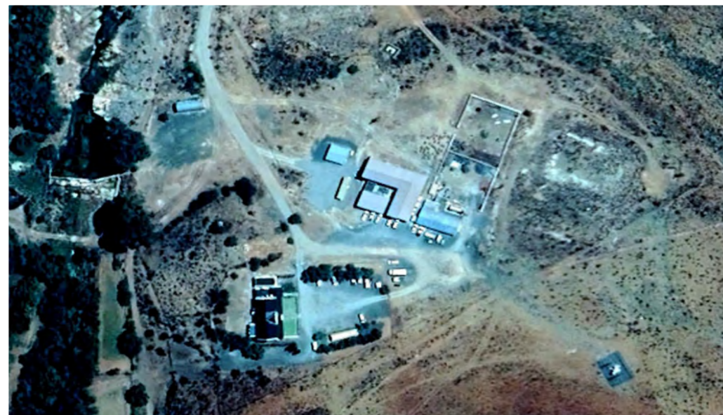
Figure 43: There have been a number of changes since the SARA0/SKA took over the site as the KSB. These include the new operations centre, temporary container offices, new parking in front of the farm house, a new gate house as well as the tarring of the road from the site leading to Carnavon. (Google Earth)
