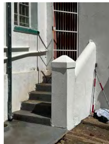
Figure 11: Steps to bathroom and server room
