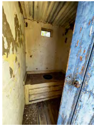
Figure 72: Remainder of long drop toilet
