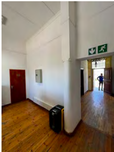
Figure 27: View of hallway from reception
