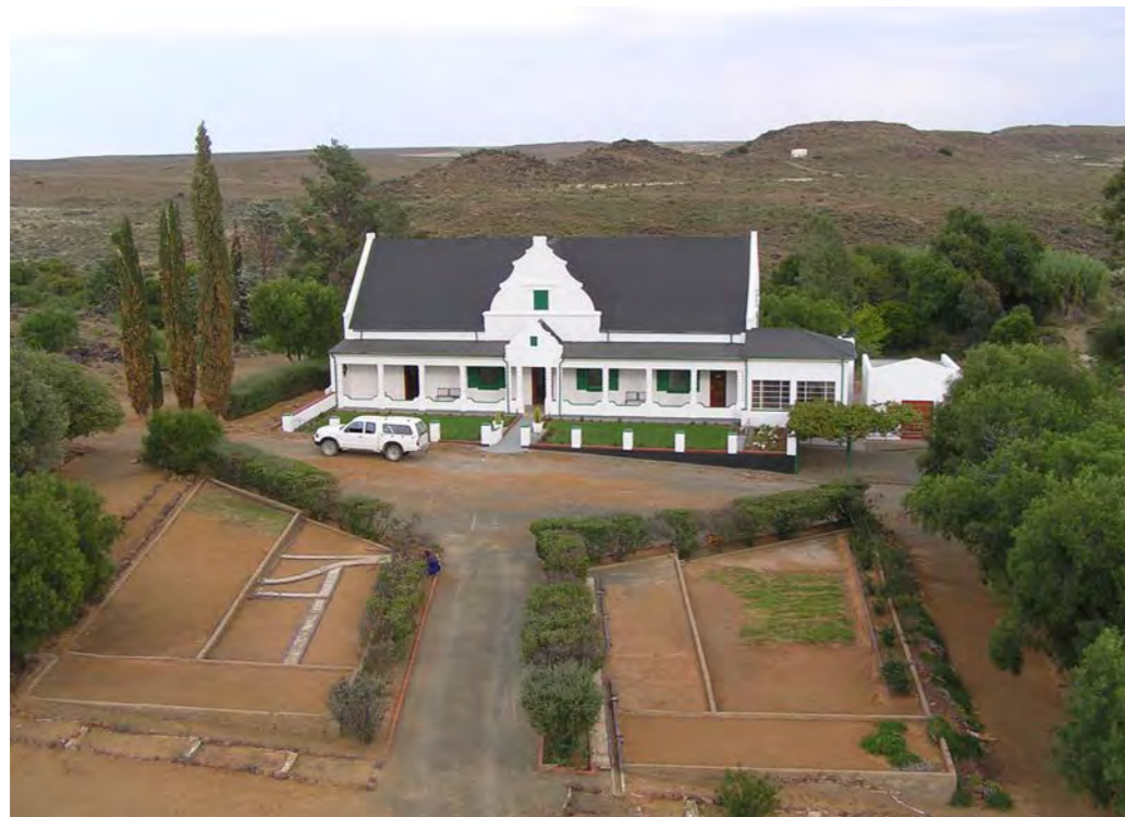
Figure 23: circa 2008 Aerial view of the werf in front of the farmhouse prior to its redevelopment as a parking lot
