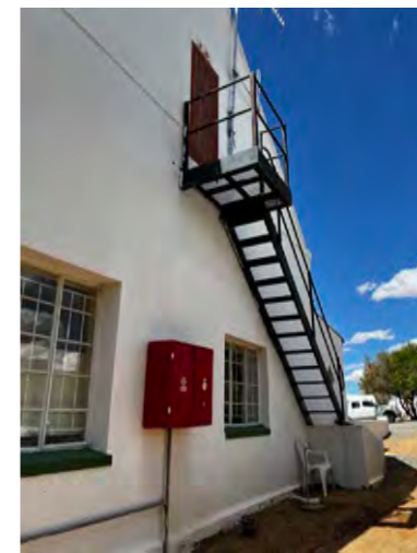
Figure 13: Stairs to loft
