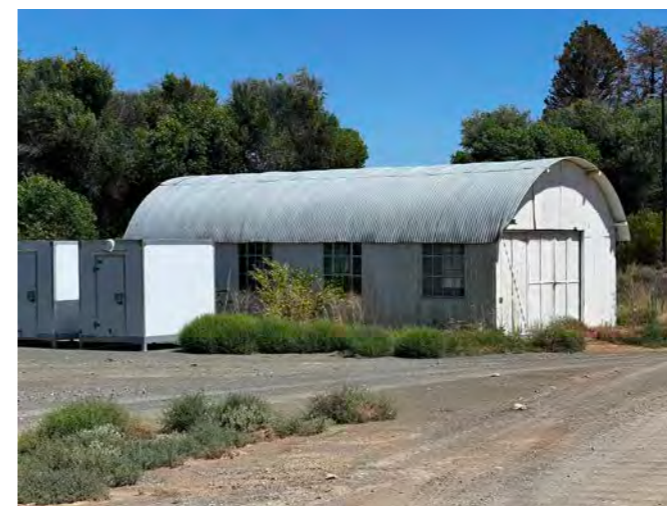
Figure 73: View of Barn
