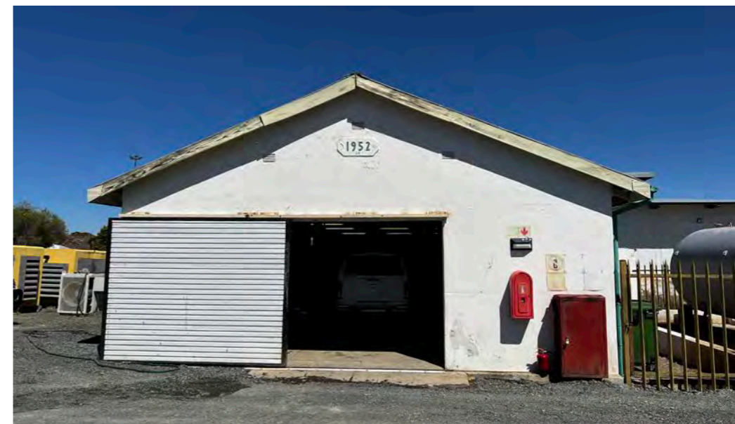
Figure 34: East elevation of the Workshop building with date of construction (1952)
