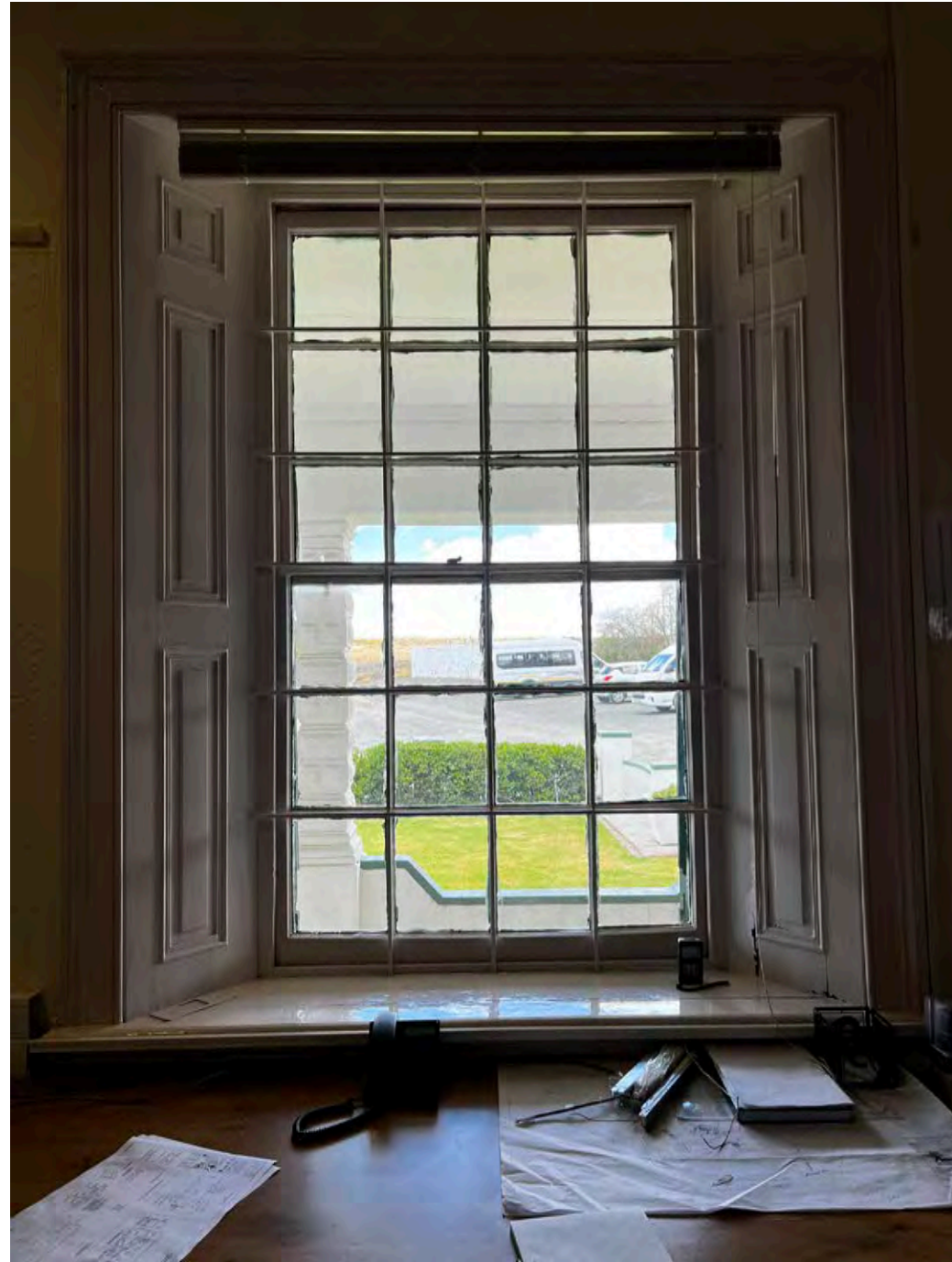
Figure 28: The internal panelling and detail of the sash windows
