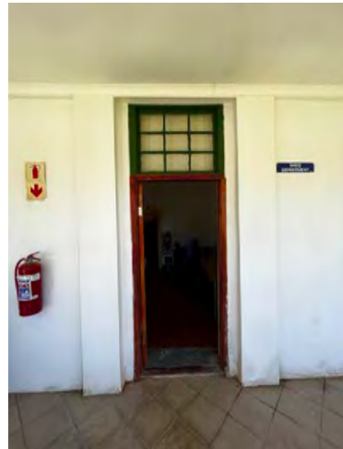
Figure 25: Front door exterior
