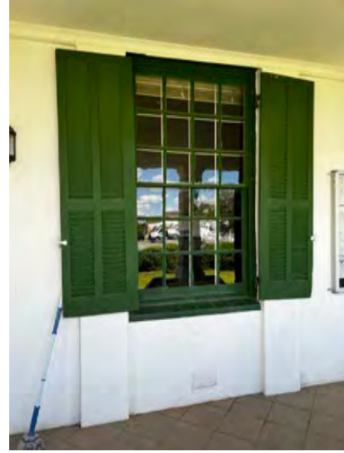
Figure 22: Window and shutters
