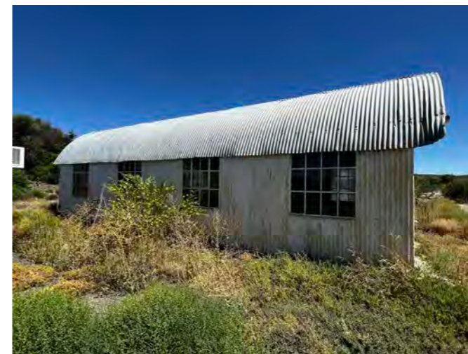
Figure 75: View of Barn
