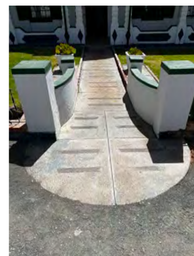
Figure 19: Entrance to farmhouse
