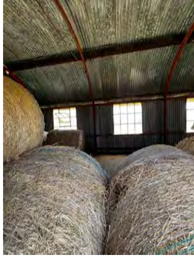
Figure 77: Interior of barn
