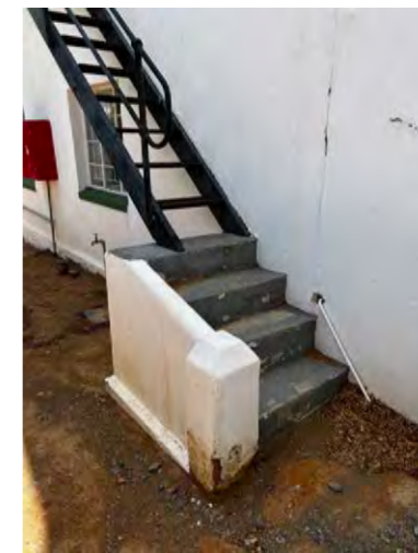
Figure 14: Stairs to loft
