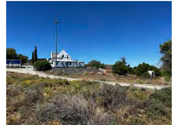
Figure 03: View of north facade from Road
