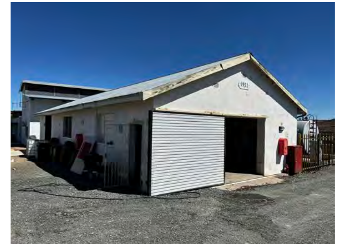
Figure 60: View of Workshop
