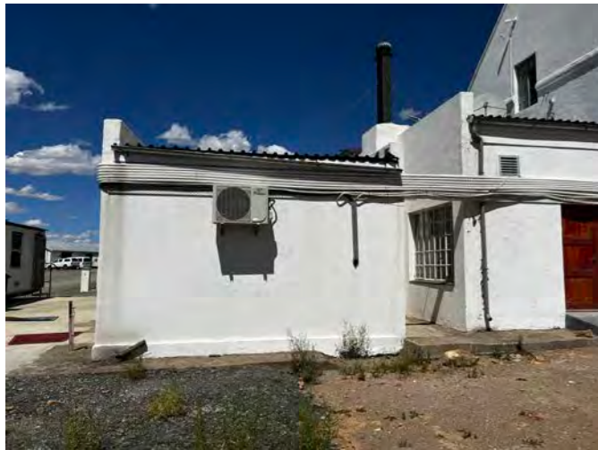
Figure 08: West Facade of garage
