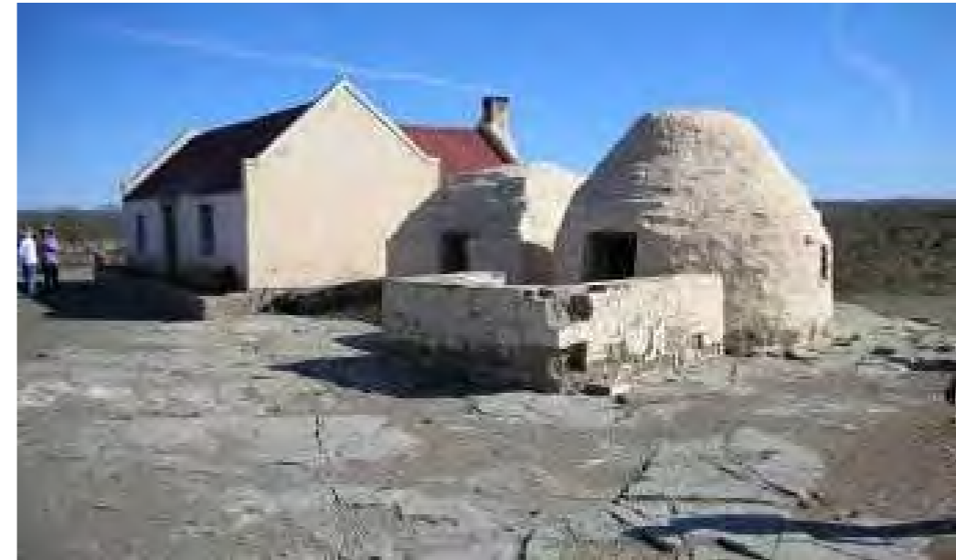
Figure 18: Vischgat homestead showing the evolution of architectural styles including circular corbelled hut, square corbelled hut and T plan pitch roof house with a brak dak buite kamer attached (VASA 2007:58)
