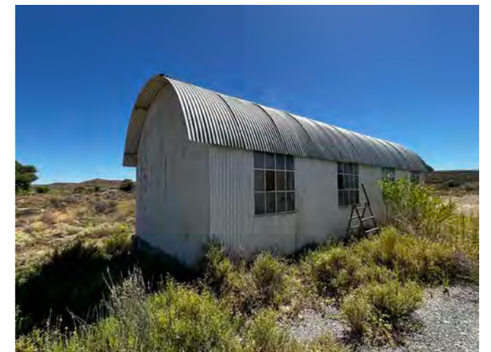
Figure 76: View of Barn
