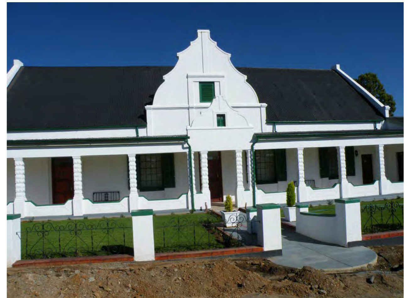
Figure 44: The farmhouse after restoration in 2010 (SARA0)
