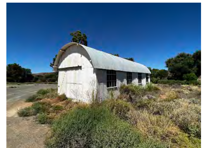
Figure 74: View of Barn
