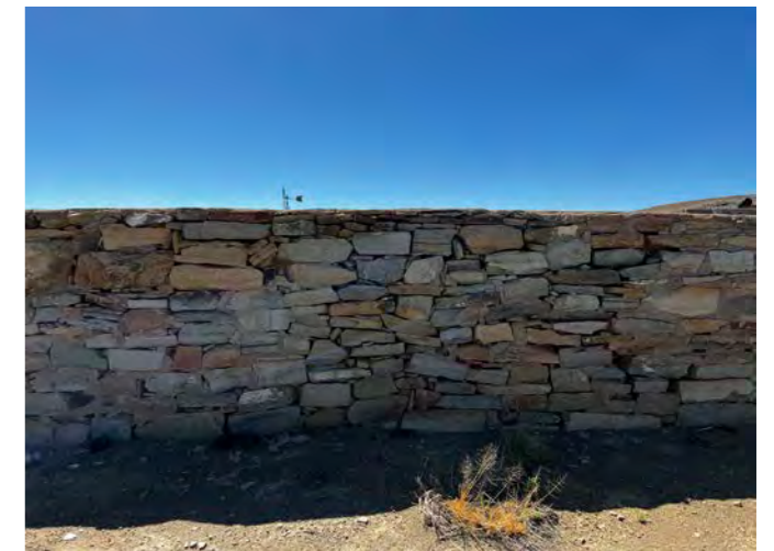
Figure 57: Stone wall detail
