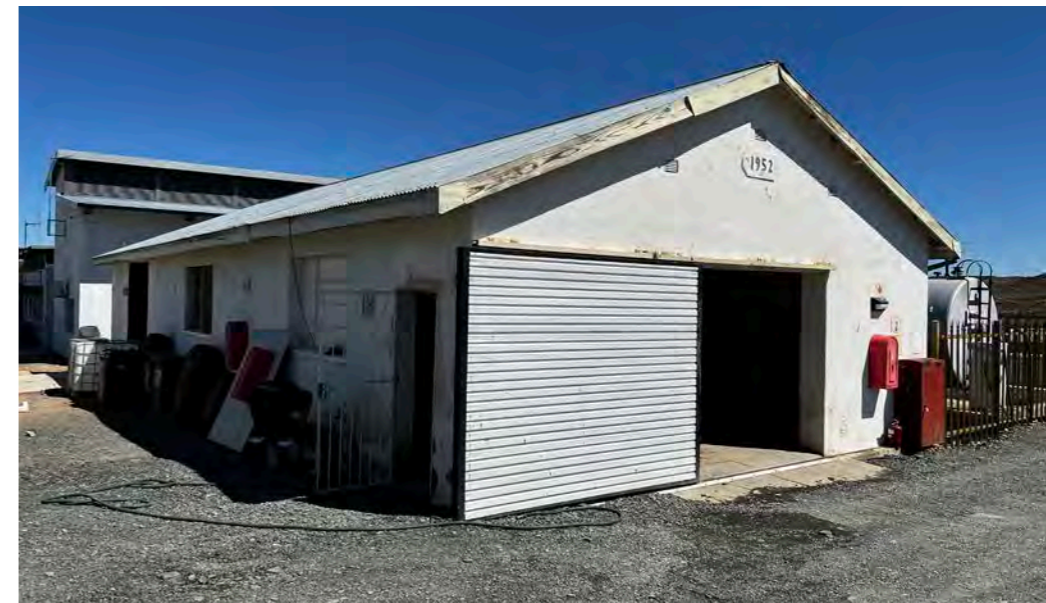
Figure 33: Photograph of the Workshop building
