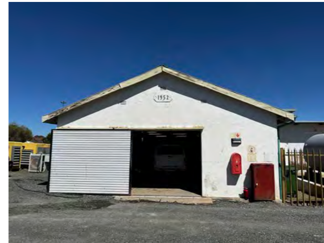
Figure 59: East facade with date
