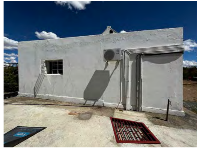
Figure 07: North elevation of garage
