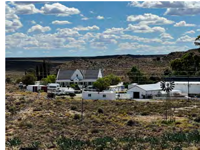
Figure 02: View of Old Farmhouse from Road
