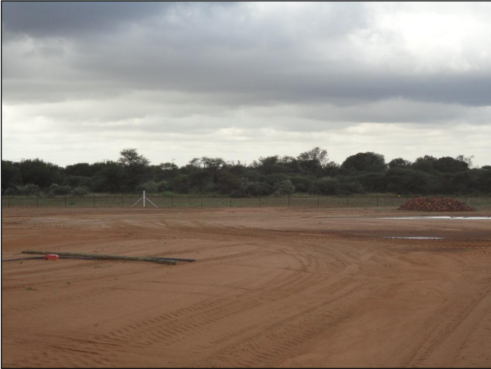
Figure 13. Eastern view of Klipparani 1
