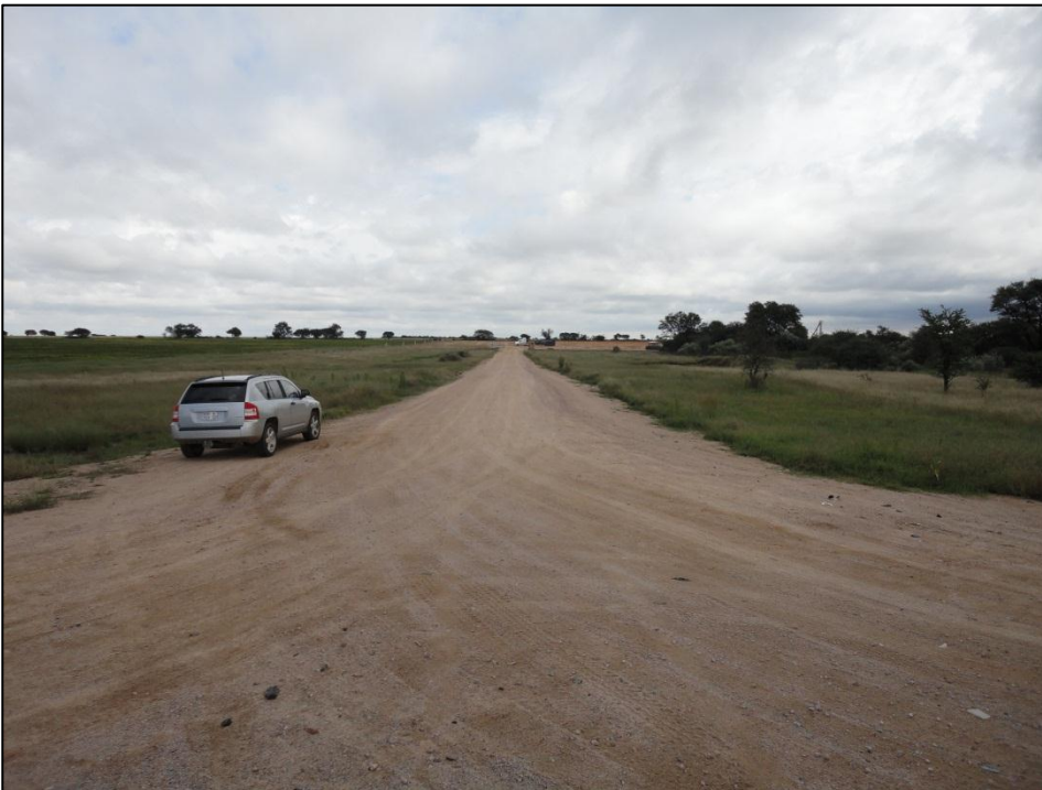
Figure 19. Existing access road to Kliparani 1 and Kliparani 2
