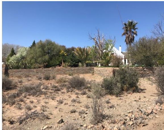
Figure 32: Close-up of the Klipkraal main farmhouse.
