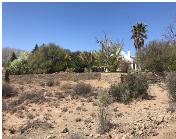
Figure 30: Close-up of the Klipkraal main farmhouse.
