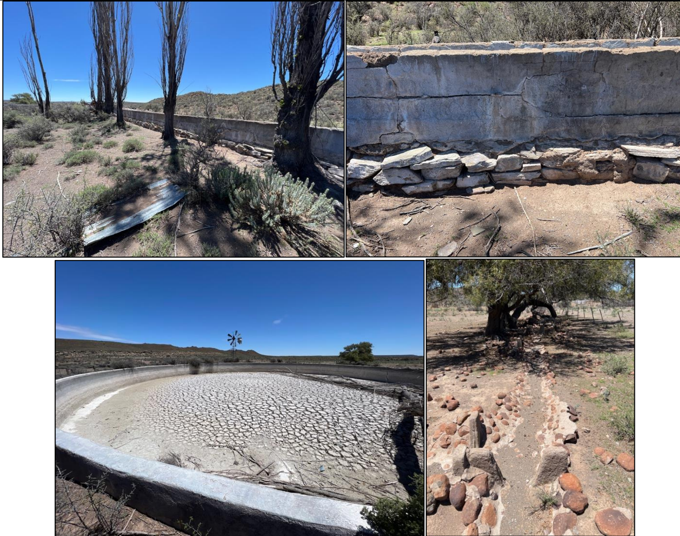
Figure 70: Views of the infrastructure identified at site 0187.
