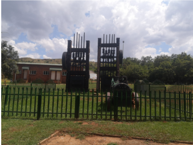
Figure 26- Struben Stamp Mill - picture taken from the north facing south. Note the engine associated with the stamp mill
