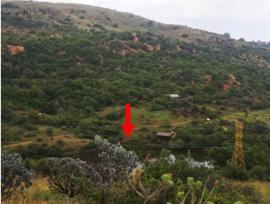
Figure 13- Picture showing the location of the dam
