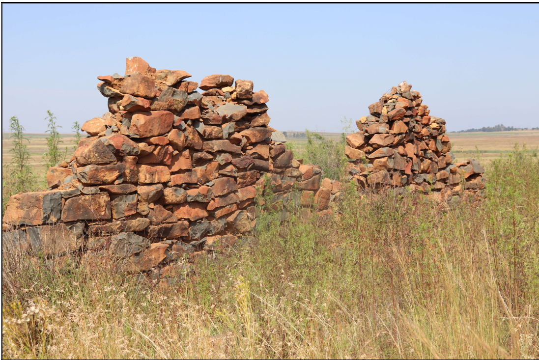
Figure 10: Stone constructed structure
