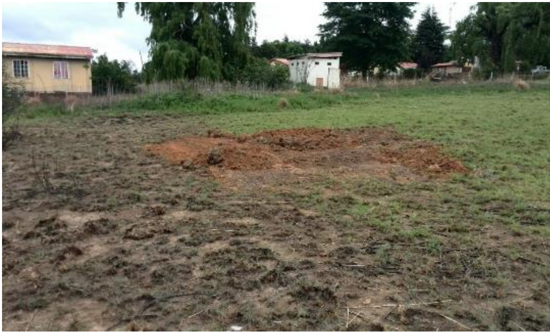
Figure 7: Recent geotechnical test pit near western boundary and residences
