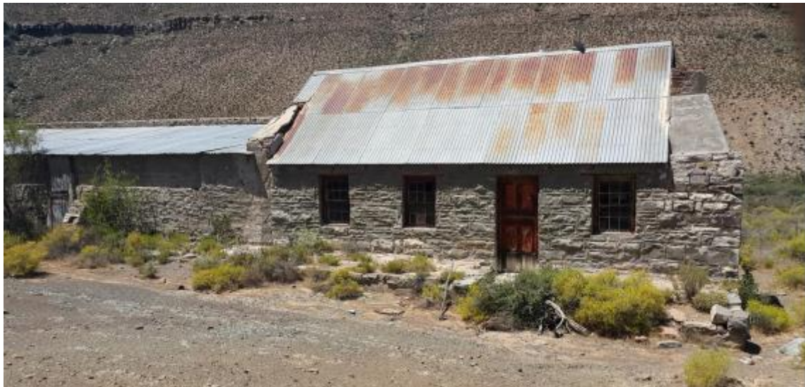
Figure 13. Farm buildings at Venters Rivier. Small 19 th century dwelling house, joinery is intact. Note the large vernacular style hearth and barn ( waenhuis ) appended onto the gable end.
