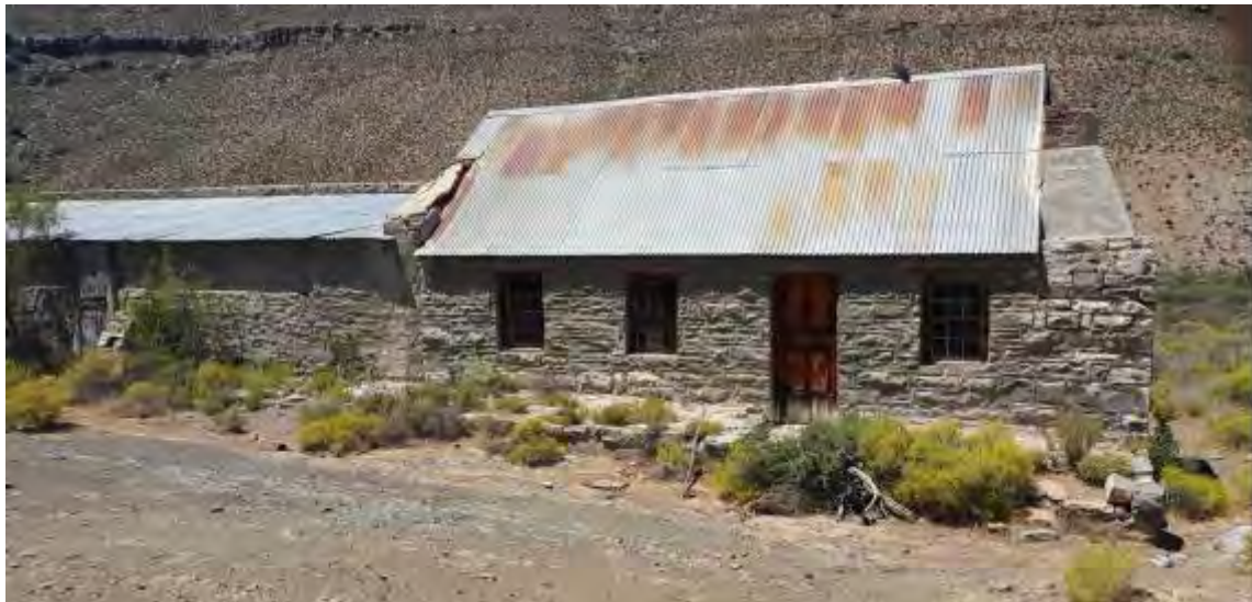
Figure 13. Farm buildings at Venters Rivier. Small 19 th century dwelling house, joinery is intact. Note the large vernacular style hearth and barn ( waenhuis ) appended onto the gable end.
