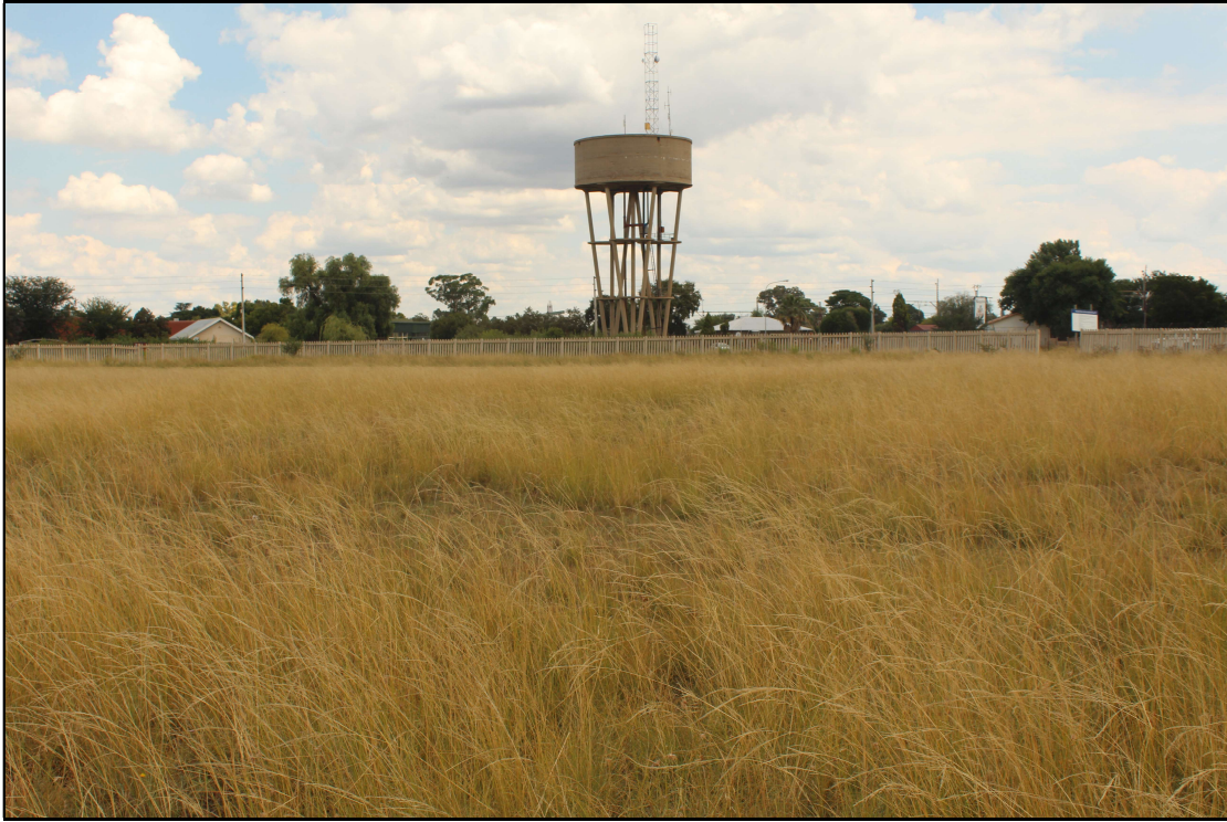
Figure 4: Raised Concrete reservoir.
