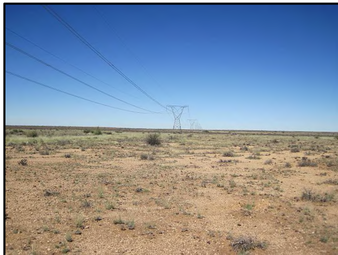
Figure 6. Existing powerlines (Aries/Helios 1 400kV).
