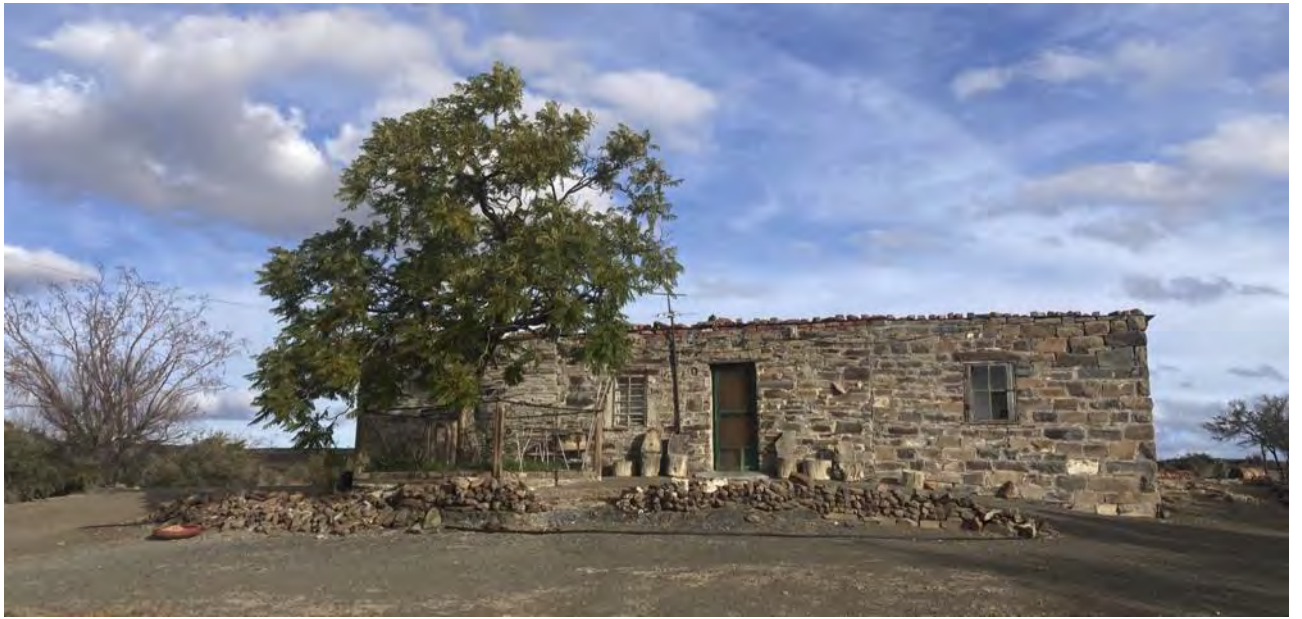
Figure 51: Kareerivier homestead front facade
