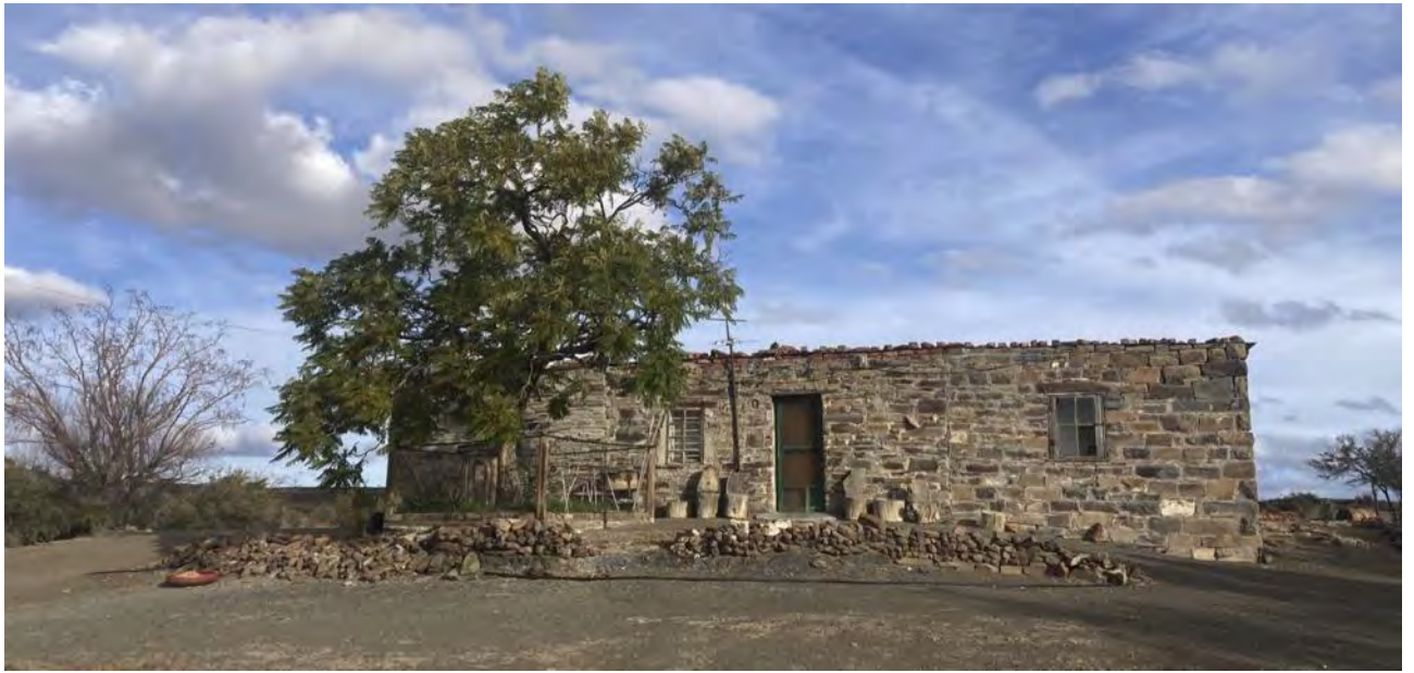
Figure 51: Kareerivier homestead front facade
