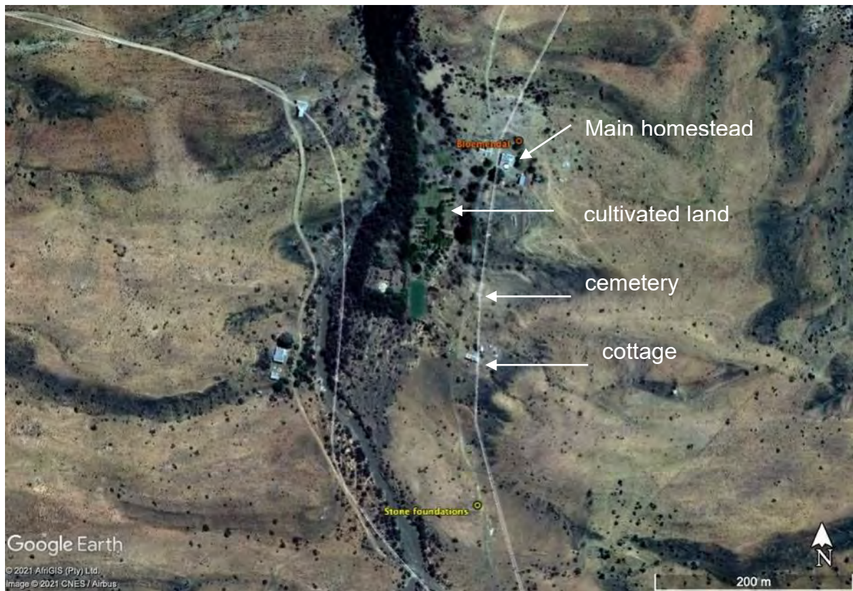
Figure 39: Aerial view of Bloemendal farmstead showing cluster of buildings, cemetery and cultivated lands in the dry watercourse and stone foundations. The stone cottage and Reynartskraal homestead (acc to the 2016 1:50K topo) across the dry watercourse.
