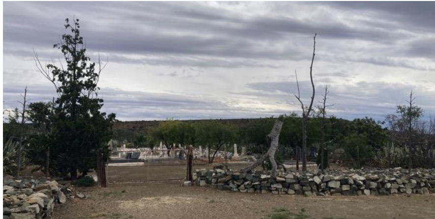
Figure 17: Examples of use of local stone for wall construction at Amospoortjie cemetery.
