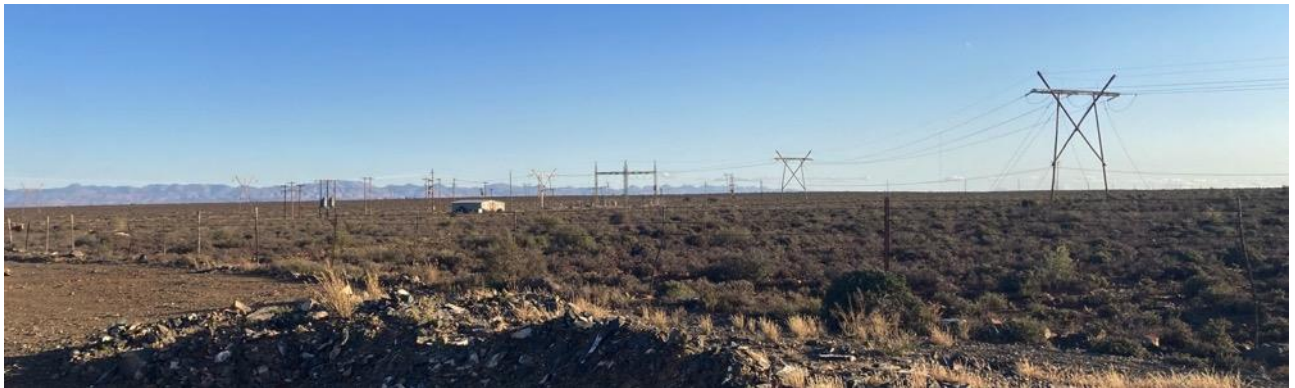
Figure 60: Industrial elements along the N12 south of the Koup landscape.
