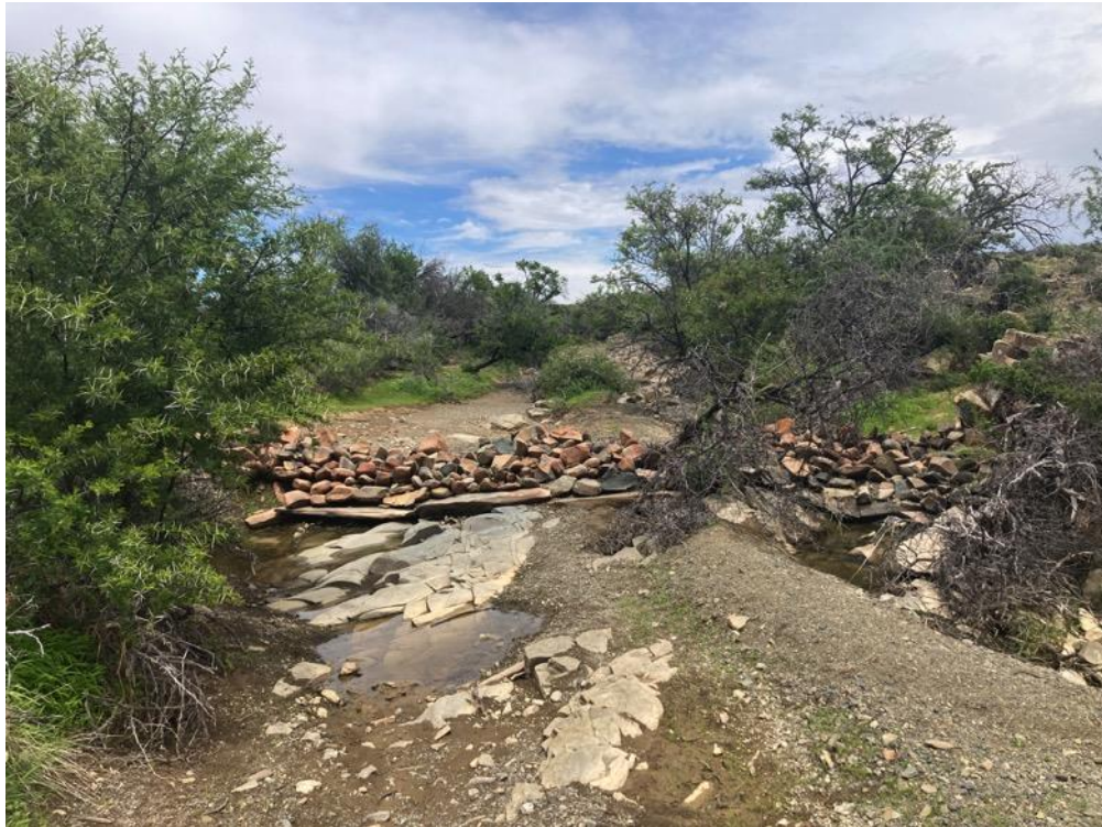
Figure 35: Kraaltjies riverine CBA adjacent showing adaptation to local natural conditions by human inhabitants through water management systems in the form of stone weirs
