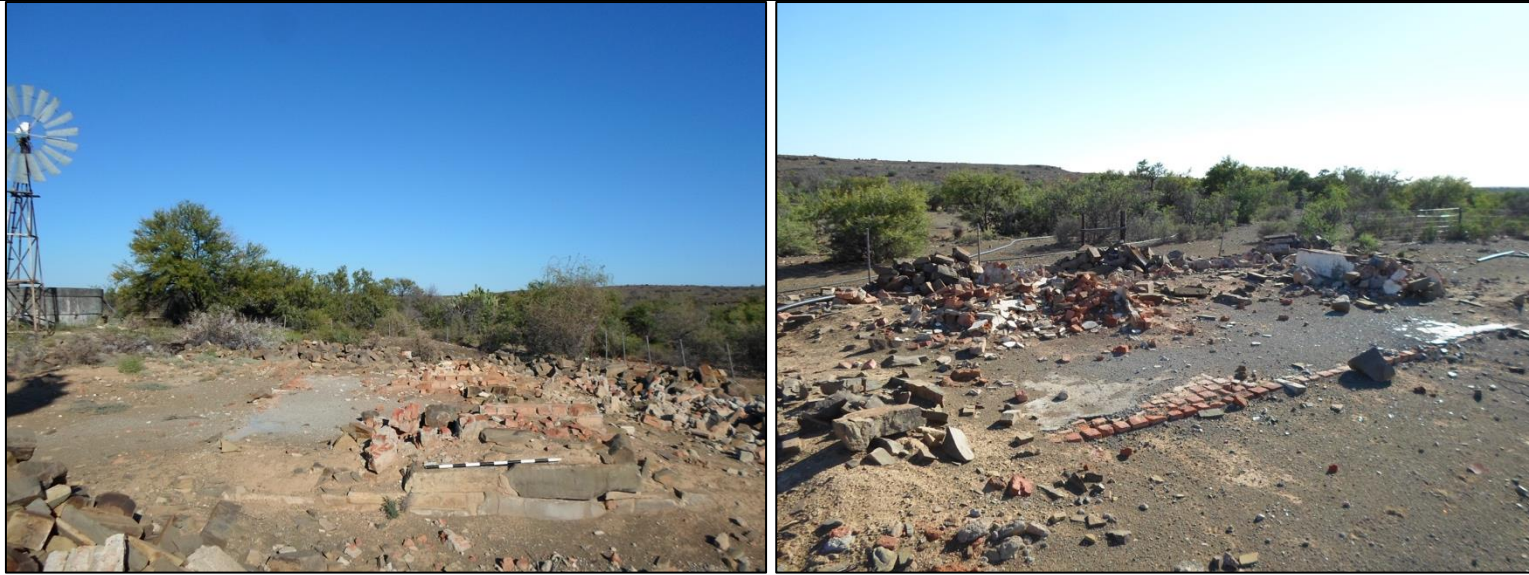
Figure 36: Views of the foundation observed at K026 near the wind pump.
