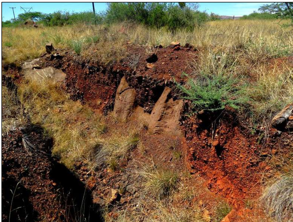
Figure 30. Deeply-karstified Campbell Rand carbonates exposed in a trench along the existing distribution line servitude south of Moffat Substation (Loc. 215). The steep-sided hollows between relict carbonate pillars are infilled with secondarily ferruginised, rusty-brown gravels of chert and BIF.
