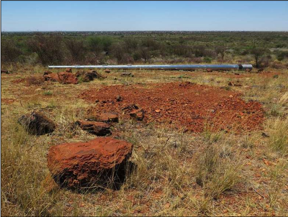
Figure 62. Example of an aluminium 132 kV distribution line monopole showing the small scale of excavation required for the pylon footing. In this region such excavations would only penetrate geologically young superficial deposits of low palaeontological heritage sensitivity (Loc. 242).
