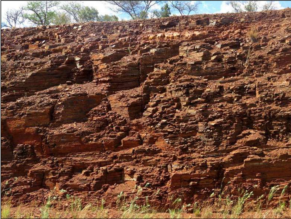
Figure 33. Road cutting exposure of thinly-bedded, tabular ironstones of the Daniëlskuil Formation (Asbestos Hills Subgroup) along the R31 between the Gamohaan and Riries Substation sites (Loc. 277).
