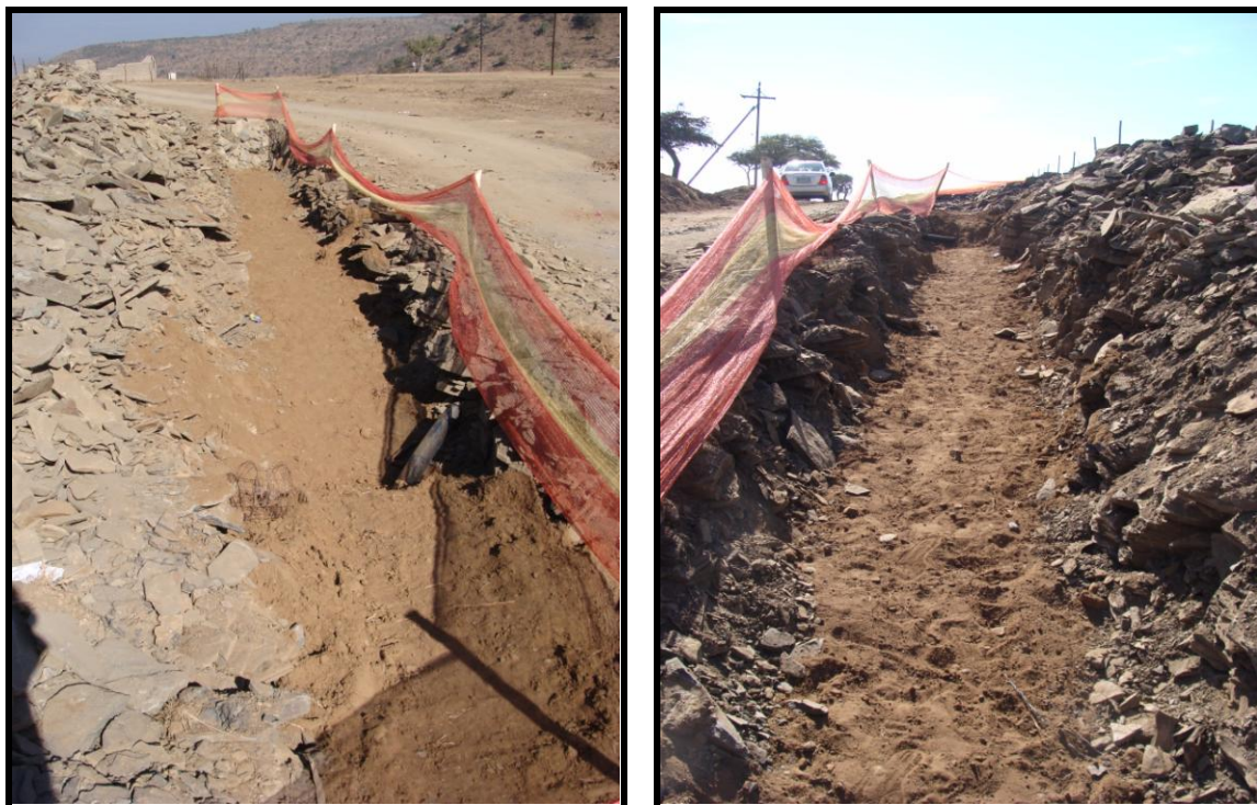
Figure 10 & 11: Pipeline trenches dug adjacent to the road leading up to iNhlabamkhosi, with piles of shale waiting to be pushed back over the trench once the pipeline has been laid and connected. These piles were examined for traces of fossils, but were dusty and unstable, making them challenging to survey.
