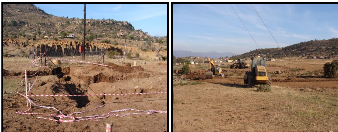
Figure 16 & 17: To the east of the R33 and adjacent to the Fabeni River, a pocket of Quaternary alluvium was exposed very close to the position of the borehole (left). A stratified sediment package is visible behind the power line pole, which contained archaeological material but no visible fossils. A construction crew were busy with heavy earth moving equipment and were busy digging into the uppermost part of the floodplain deposit, a unit which is likely to contain abundant lithic material
