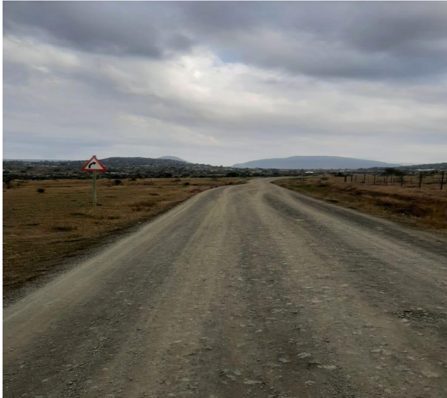
Figure 17: View of a dust road in the in Phalafini area
