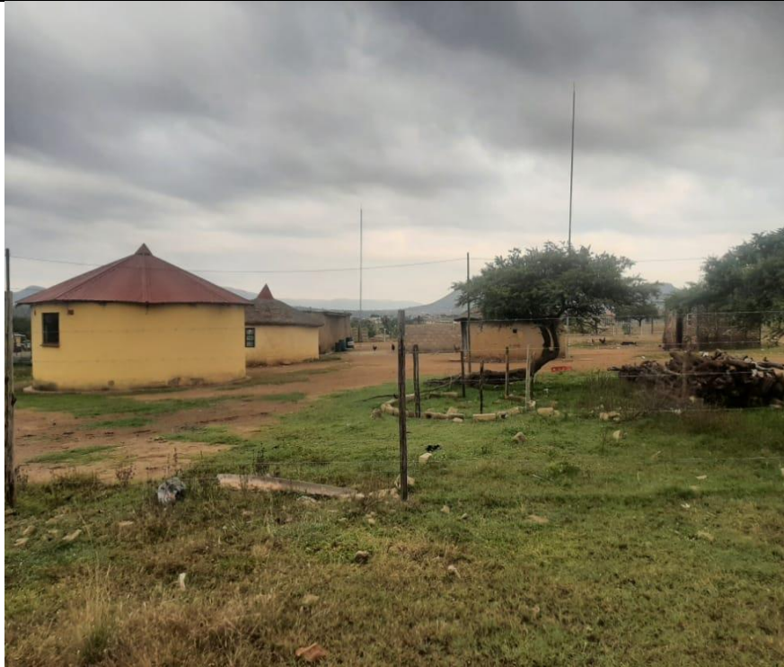
Figure 19: Typical rural homesteads around the proposed development footprint
