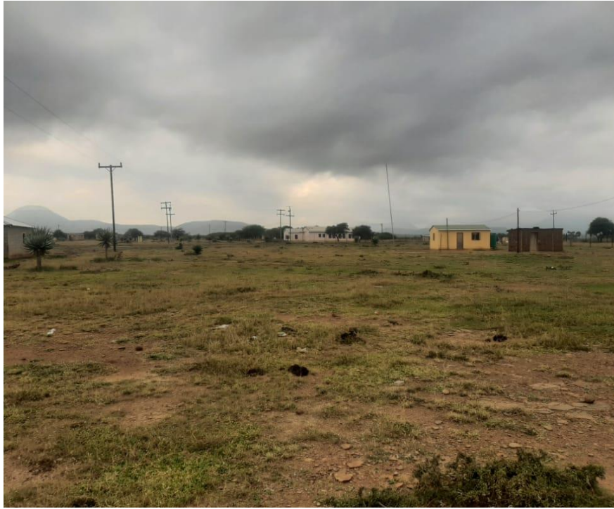
Figure 15: View of electricity power lines traversing across the proposed development site
