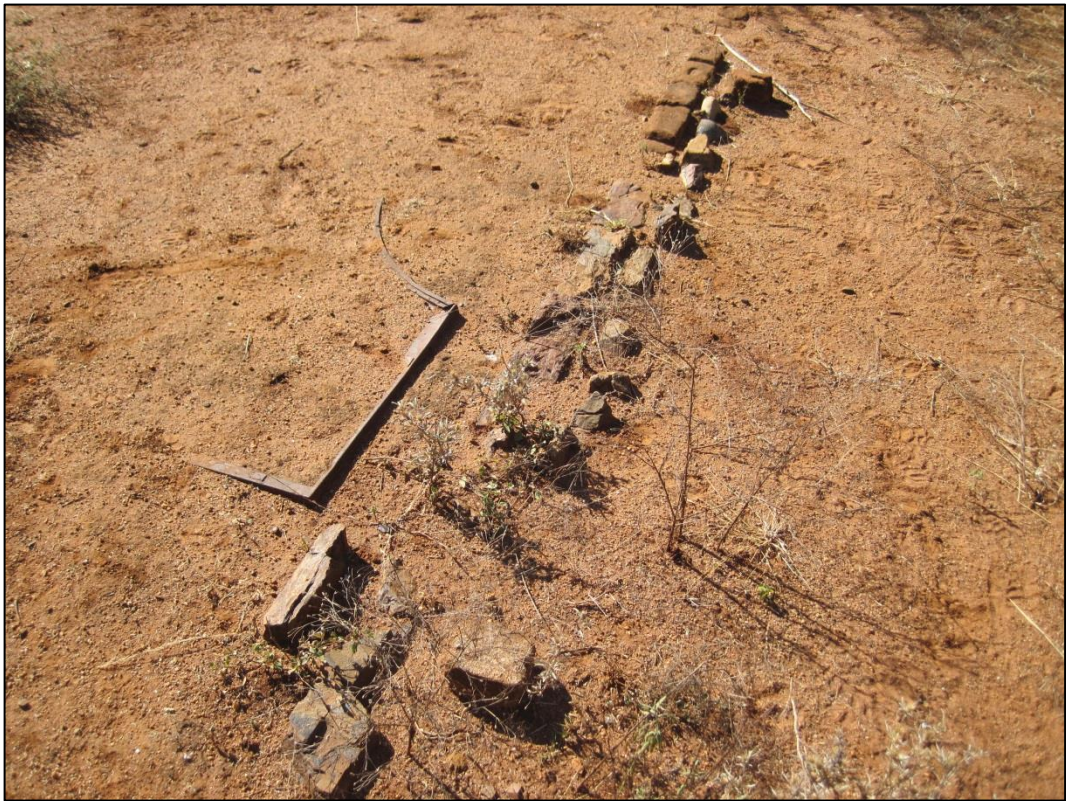
Photo 8: View of the double line foundations of the structures.
