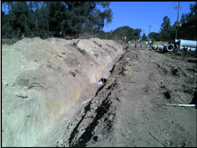
Figure 7: Pipeline trench on the western boundary of the study area.
