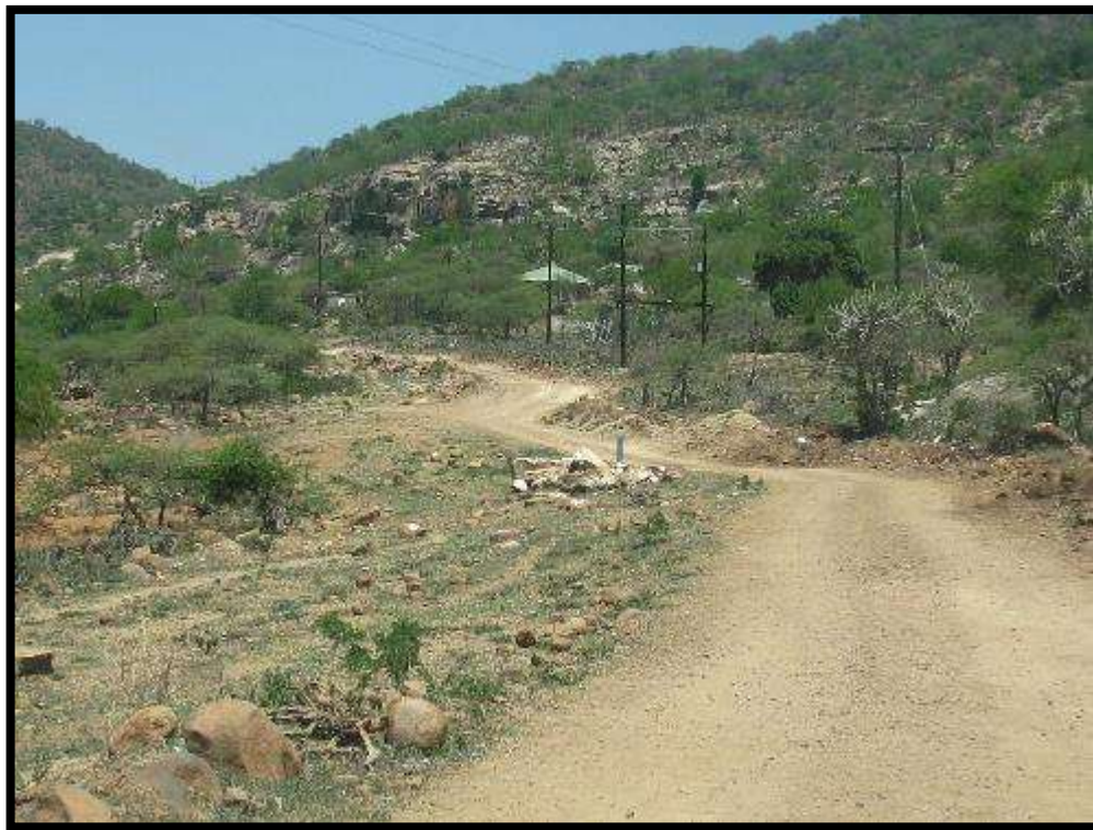
Figure 7. View of the L1859 extension.
