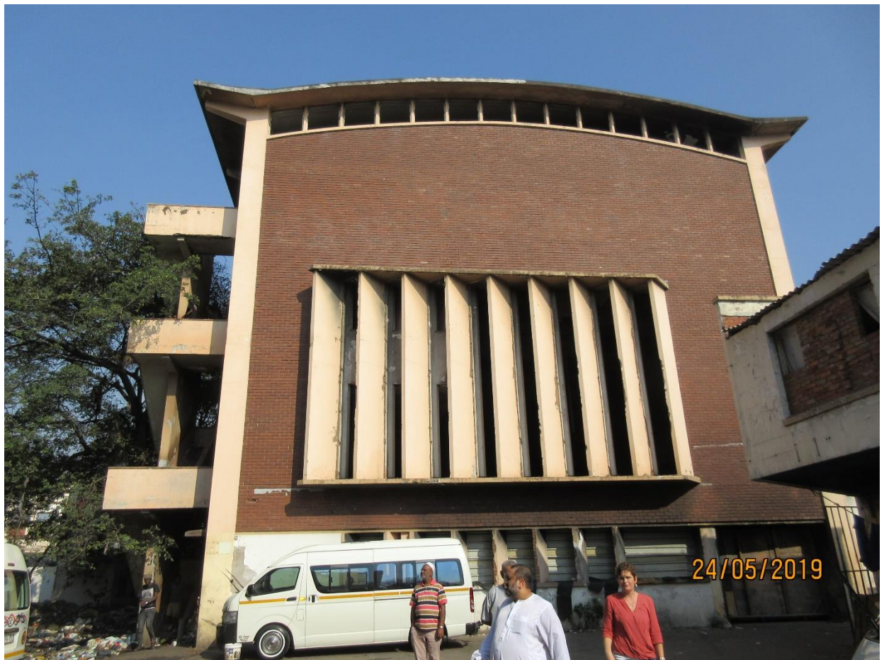
Figure 9: North-eastern façade in May 2019. Source: Prof Walter Peters
