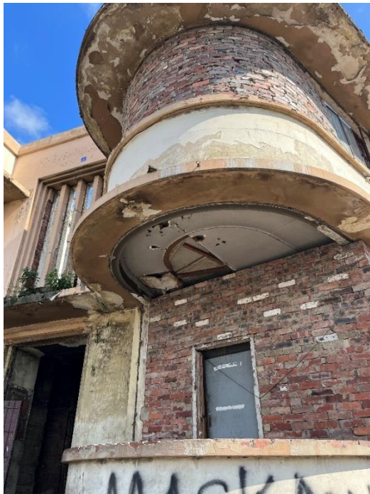
Figure 12: Infill brickwork inserted into the main entrance, May 2021.
