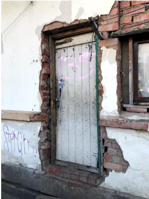
Figure 10: A door inserted into the University Ave façade, May 2021.
