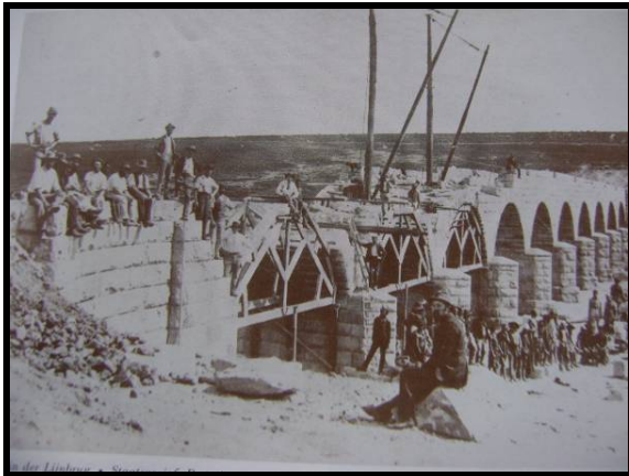
“Begin der Lijnbrug” bridge during construction Photograph: Transvaal Archive
