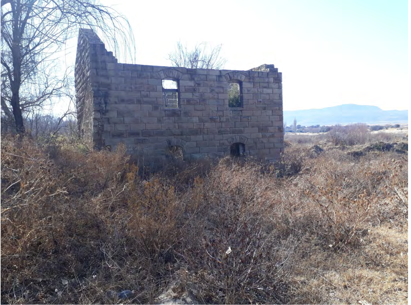
Figure 16. Remains of the old mill, looking north towards the old bridge crossing, located near but just outside the north-eastern boundary of the mining right footprint and about 300 m away from the proposed mining area.
