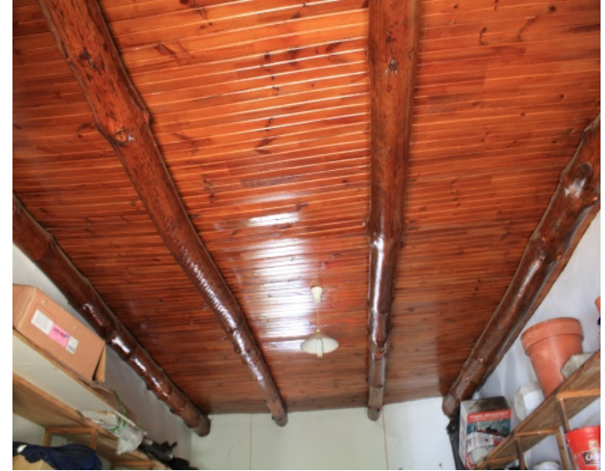
4.2.6 Pine ceilings in spaces between garage and stables
