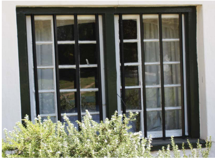
4.2.5 Typical double casements c 1912
