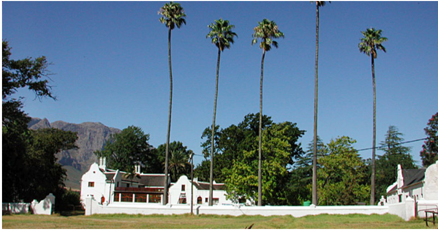
4.1.1 View across the werf looking southwards towards the rear of the homestead with the barn located to the far right
