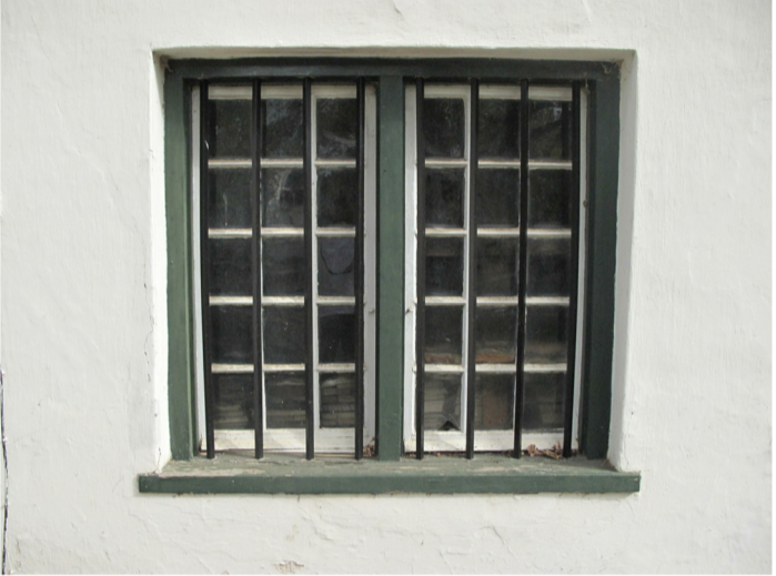
MAINTAIN/REPAIR AND MATCH EXISTING WINDOWS
