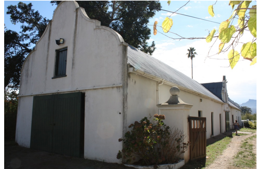
4.1.4 South-east facing front elevation and south-west facing gable end of the barn; the section affected by the proposals includes, left to right, the garage, a storeroom, a second storeroom and the coach house
