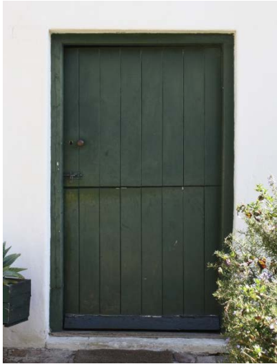
4.2.4 Typical stable doors on south-east facing front elevation
