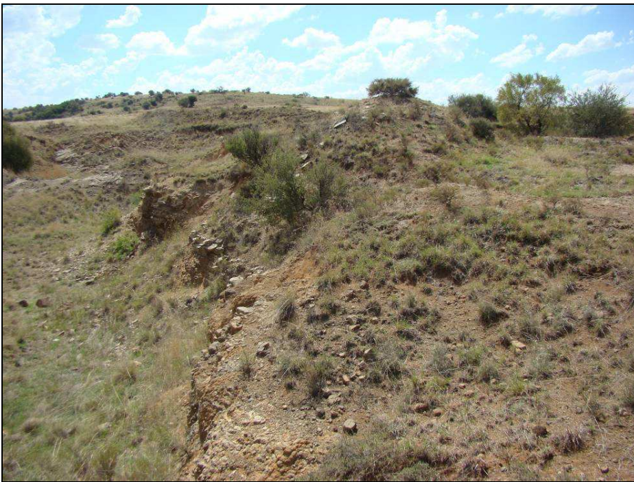
Fig.11 Borrow pit at Point E, Leratong & Tsepong near Thaba Nchu.
