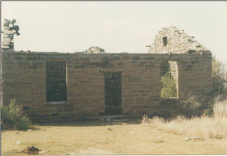
Fig.16 Sturdy old building at the Modder River pump station.
