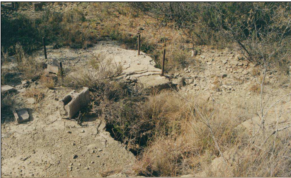
Fig.15 Fixtures for the steam engines in what used to be the pump house at Modder River.
