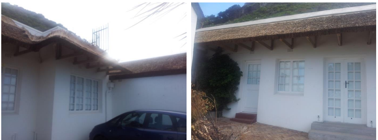
Figure 8 (left): view of “skirt” with thatched garage at Rhodes’s Cottage to RHS. Figure 9 (right): “skirt’ with flashing complete
