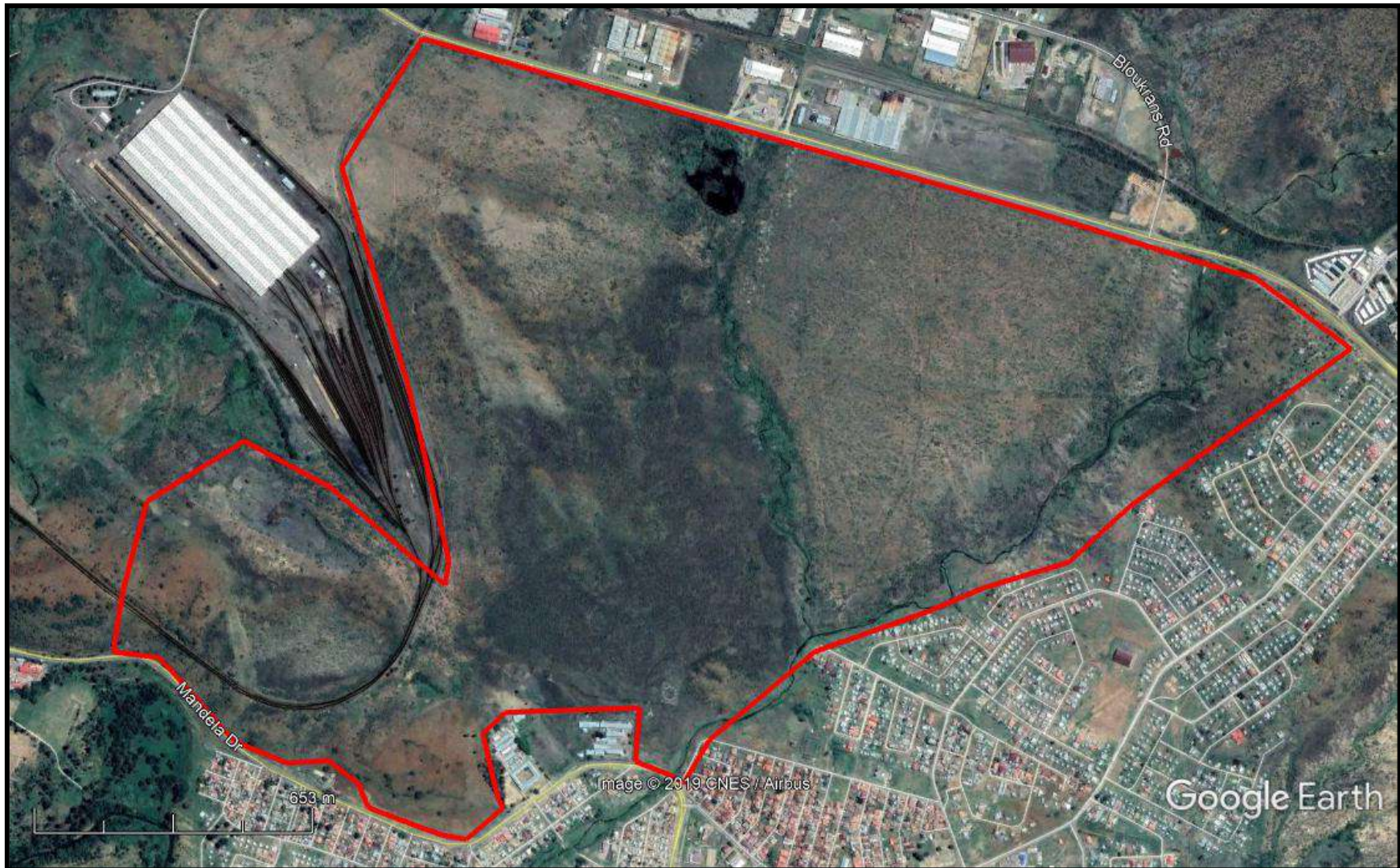
FIG. 2: AERIAL OVERVIEW OF THE PROPOSED DEVELOPMENT
