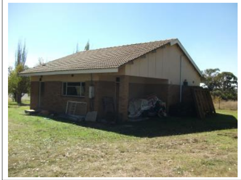
Figures 14 & 15- Two former residences in the Project Area date from the recent past and have no heritage significance. These residences may be incorporated in the Lake Umuzi South Bank Extension project (above and below).
