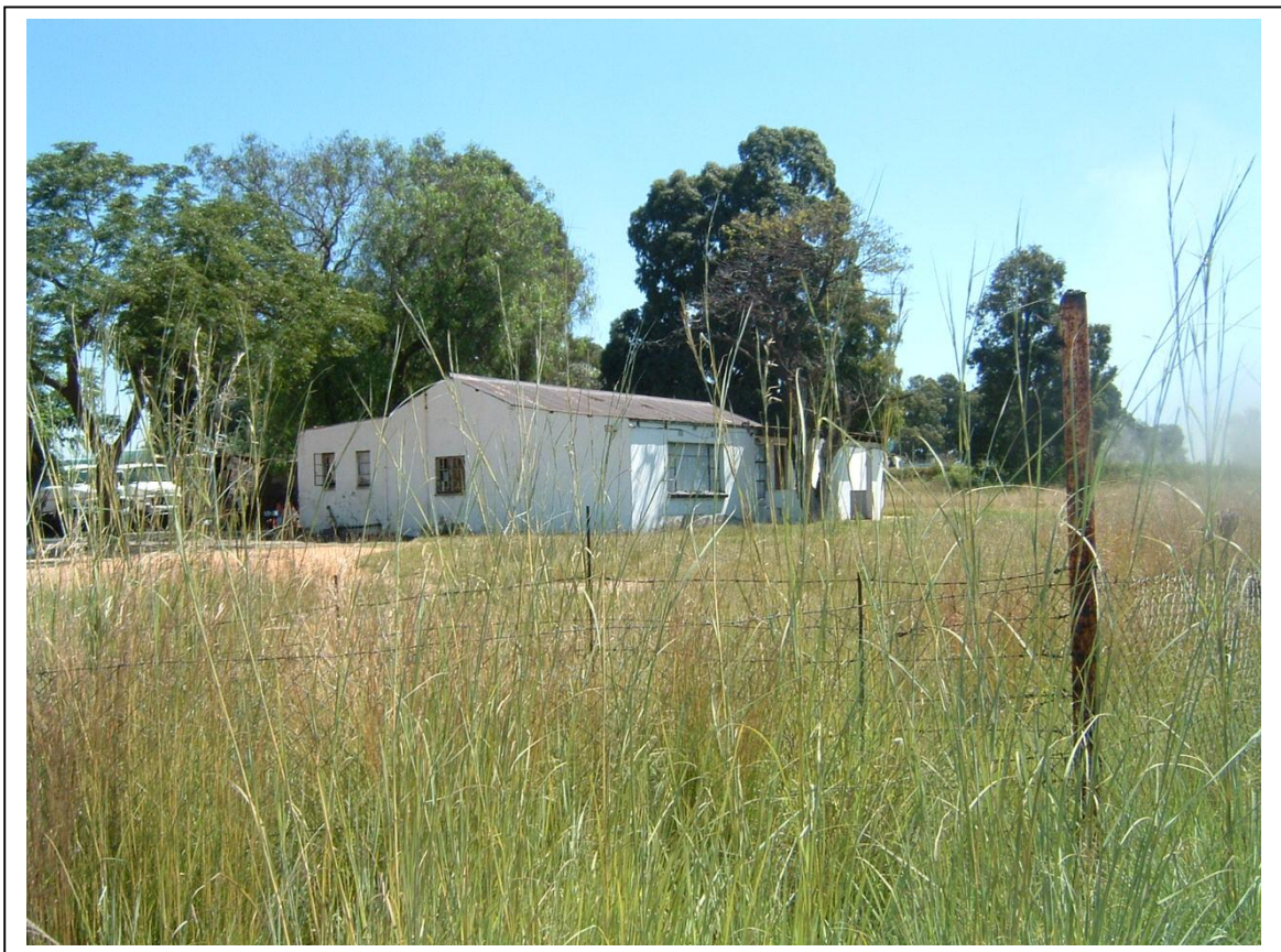
Figure 9- HH01 is located on the southern shoulder of the R104. It comprises a colonial styled dwelling which may date from the early twentieth century- or even earlier - although it has been renovated in the more recent past. This dwelling is currently still occupied (above).
