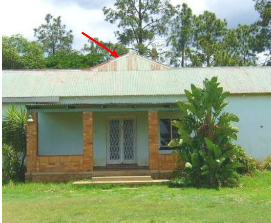
Fig 13. Site 7. Old farmhouse. Note roof structure indicating age older than 60 years.
