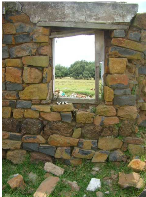
Fig. 12: Detail of a wall with the local stone clearly visible.
