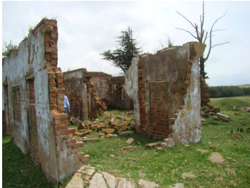
Fig. 11: Ruin of farmhouse. The original structure was built with local stone and later new additions, with fired bricks, were added on.
