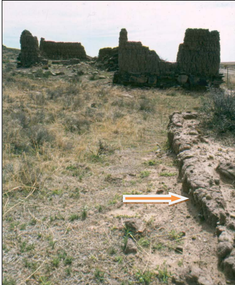
Fig. 26: The foundation of House 2 ( H2 ) in the foreground, 1986. (Photo: Jakkie Pretorius, NALN, Bloemfontein)
