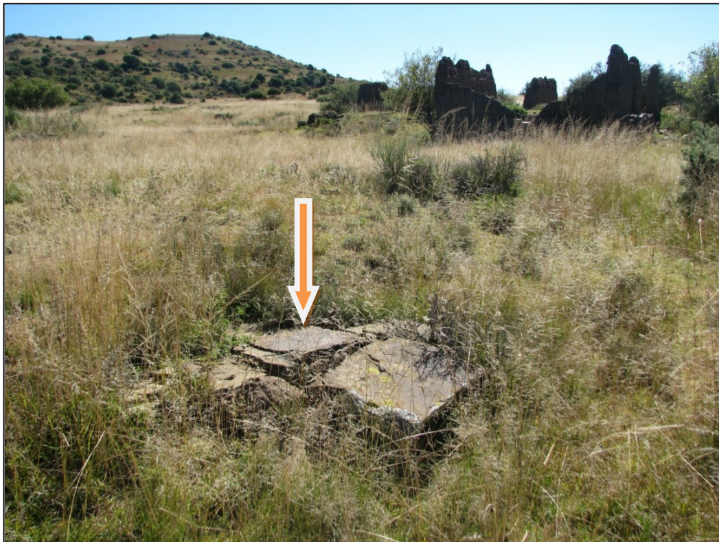
Fig. 25: The foundation of the entrance at House 2 (H2) is still visible in the grass.
