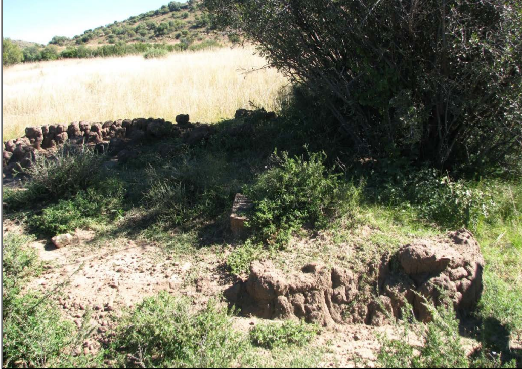
Fig. 32: Basically nothing remains of House 4 (H4), 2015.
