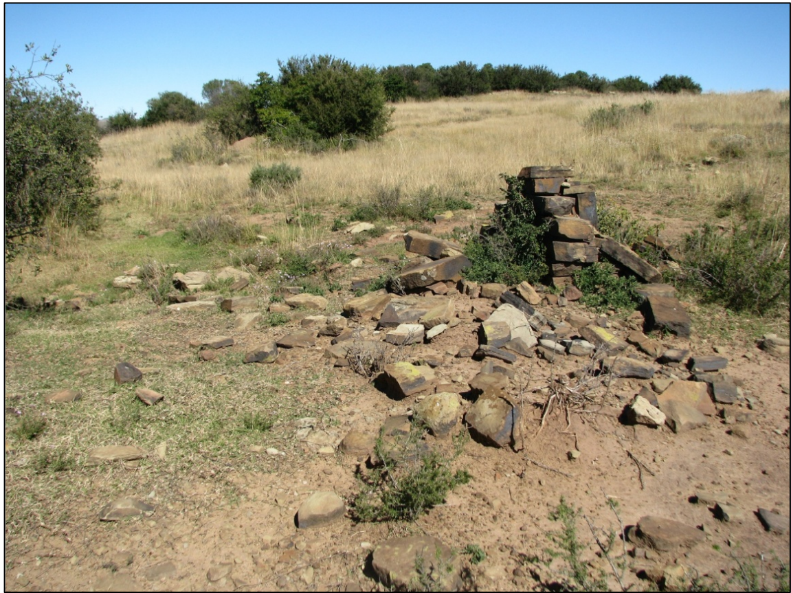
Fig. 41: Foundation of Structure 3 (S3).
