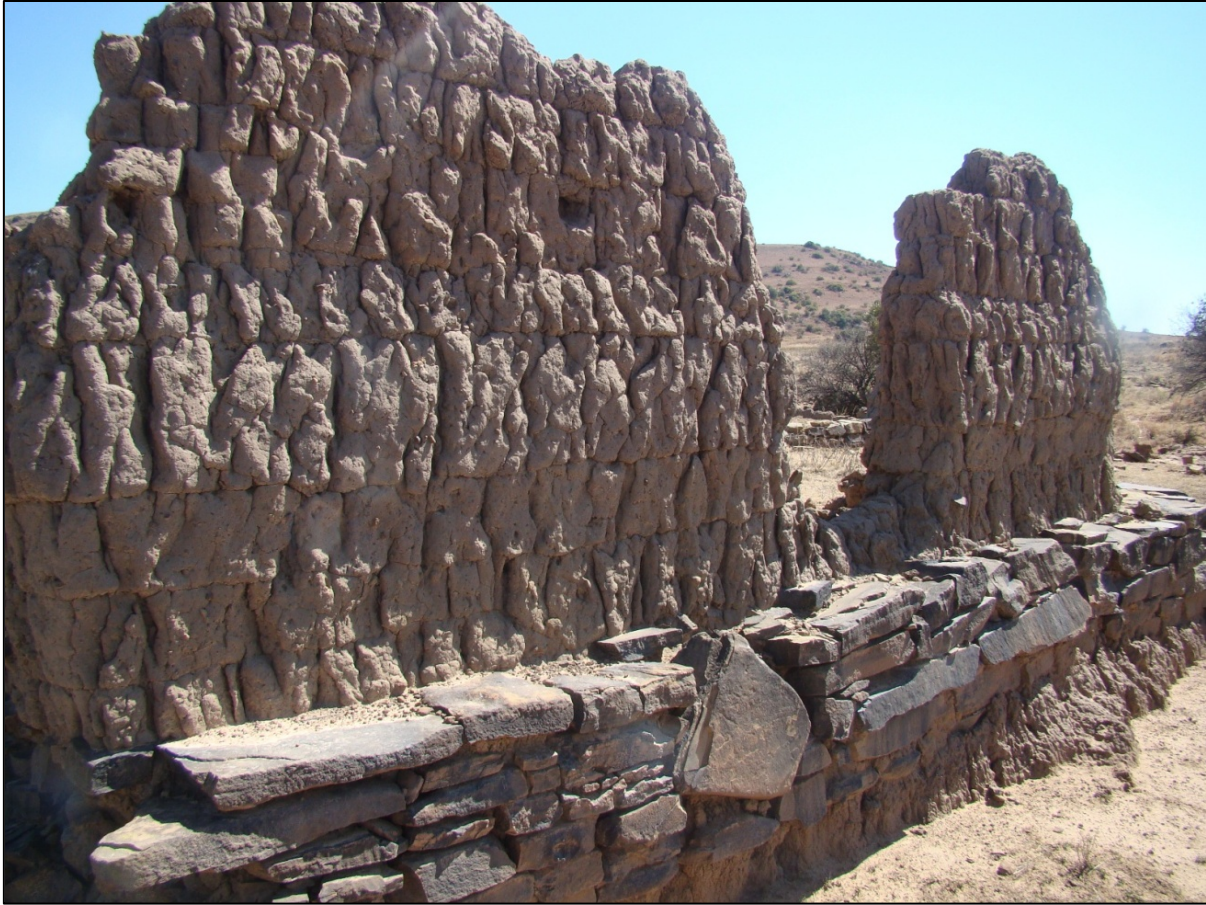
Fig. 22: Mud layered walls on a stone foundation.
