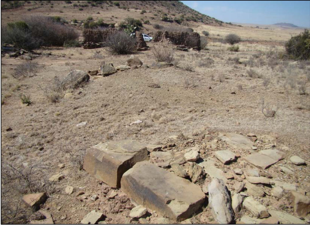
Fig. 38: Foundation of Structure 2 (S2) in the front, and House 1 (H1) in the background.
