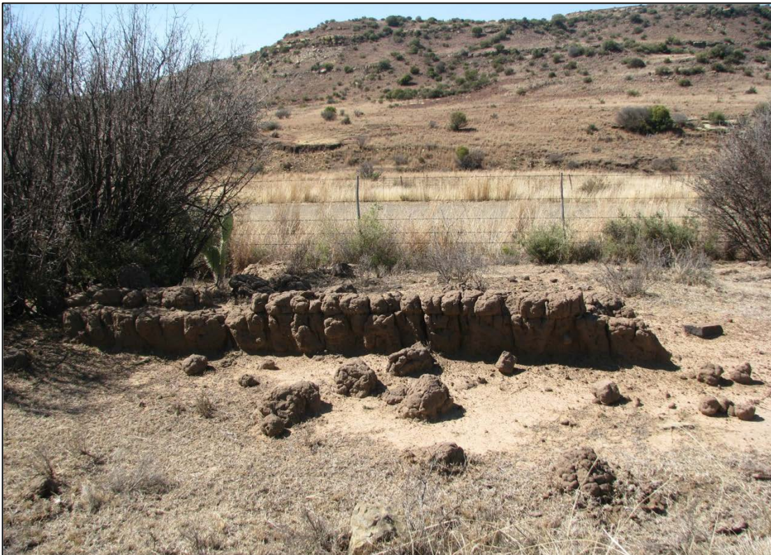
Fig. 33: Basically nothing remains of House 4 (H4), 2015.
