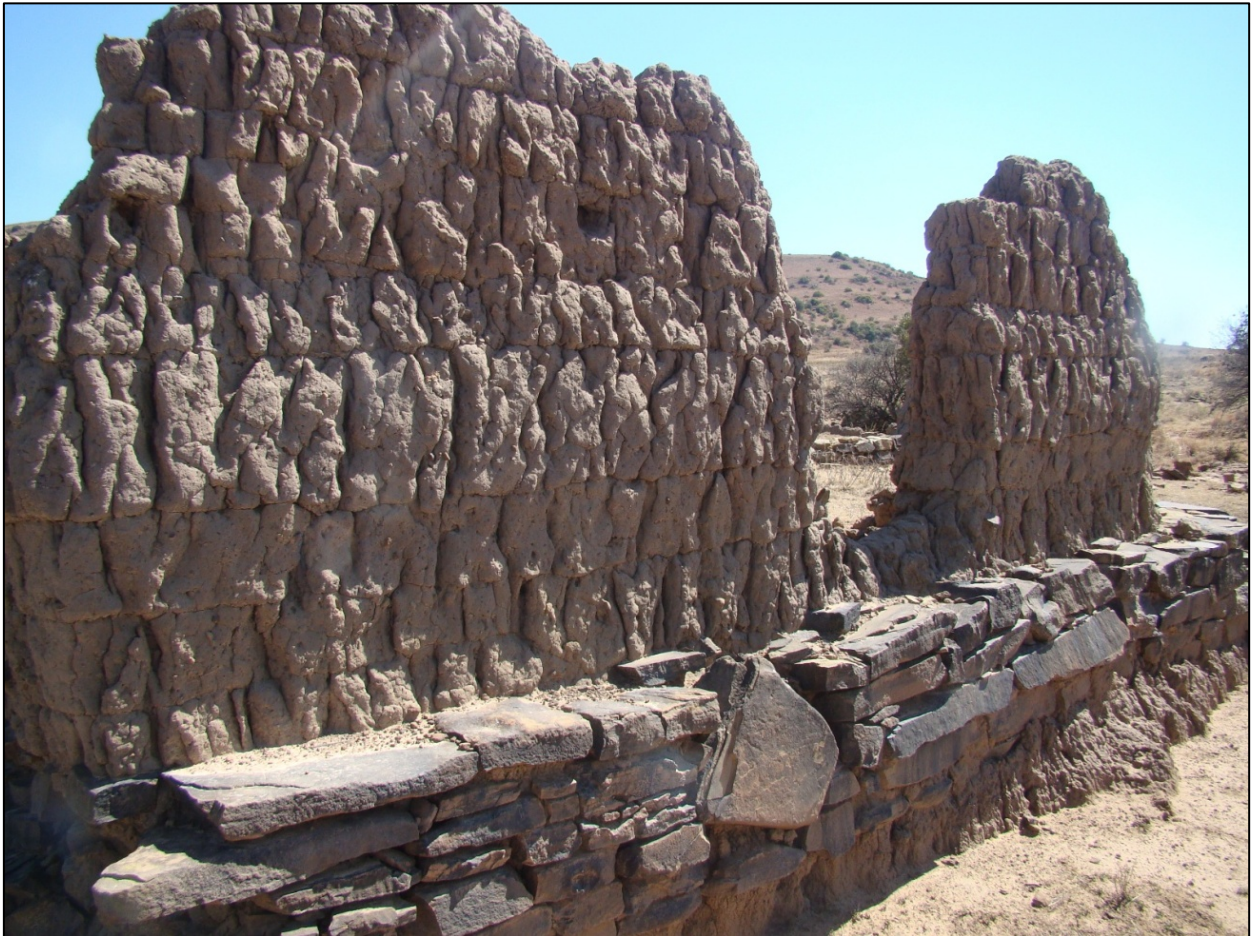
Fig. 17: Mud layered walls on a stone foundation.
