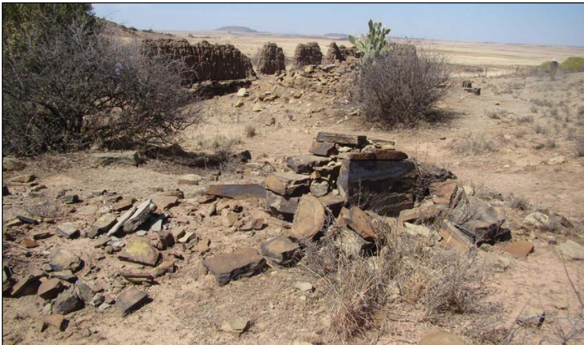
Fig. 26: The foundation of Structure 4, and House 1 in the background.
