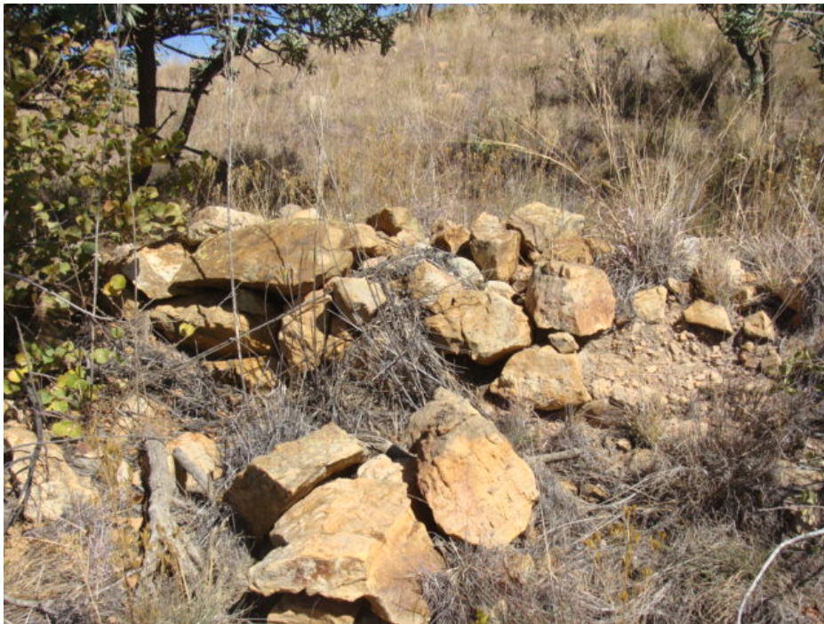
Figure 20: Military stone walling at site no. 5.
