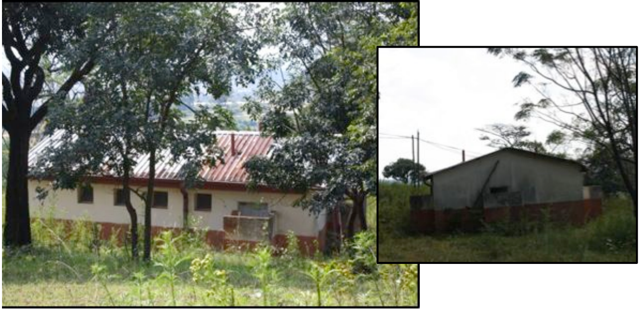
Figure 30. Bathroom earmarked for demolition
