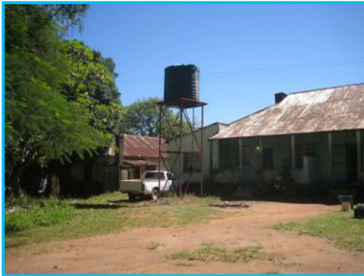
Figure 2: Water pumped from the borehole to the elevated tank located at the site
