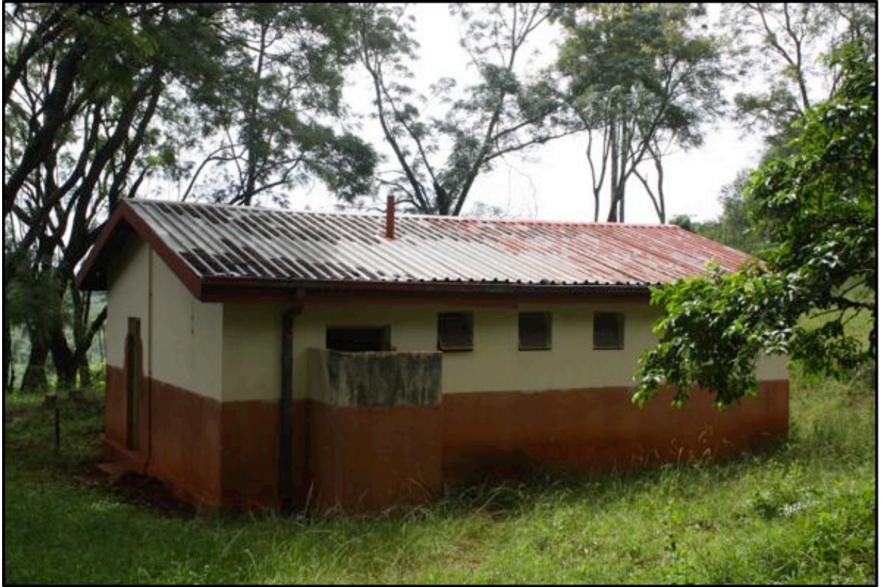
Figure 34. Ablution block to be demolished
