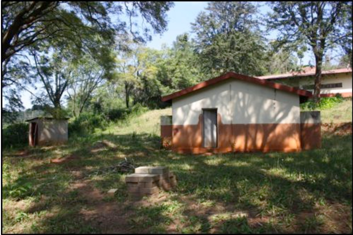
Figure 35. This structure to be demolished for new classrooms
