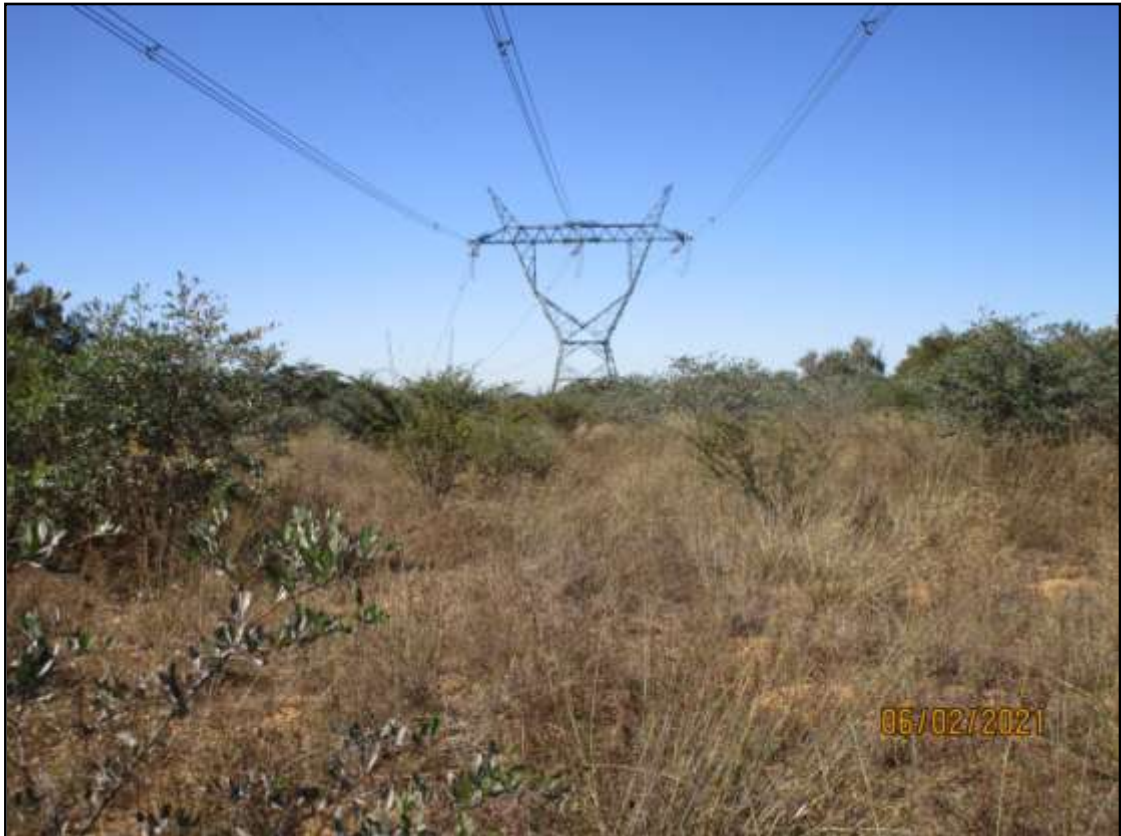
Figure 6. View of high voltage power line just east of the project area.
