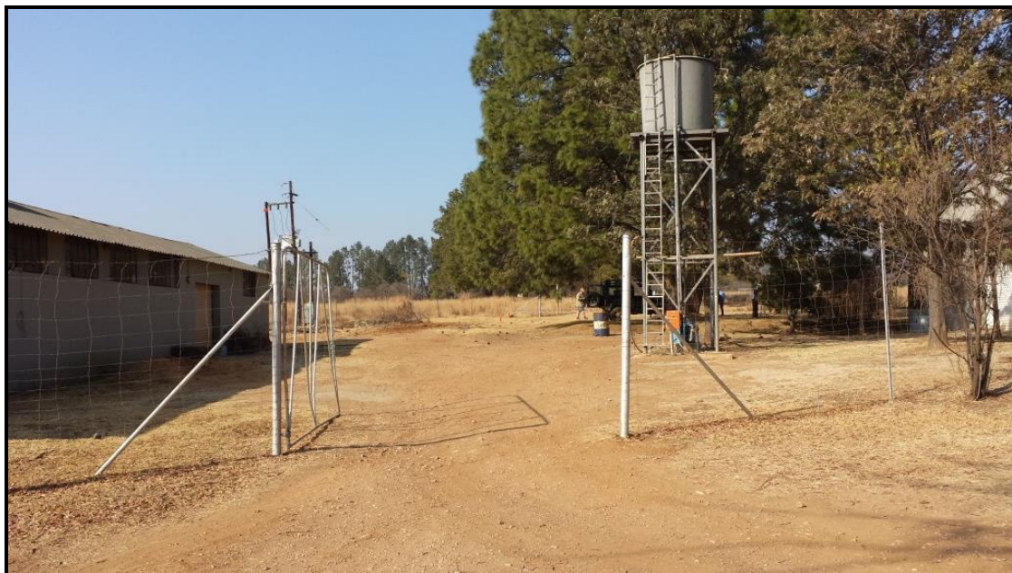
Figure 3: Existing Elevated structures in the study area.
