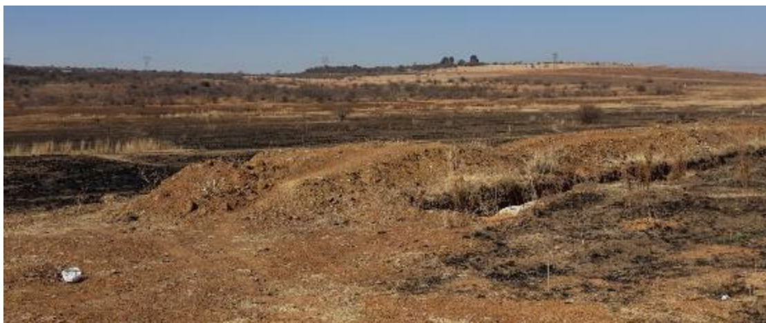
Fig. 65. Looking south from marker 7. Construction work ongoing. (Photo S.M. Miller 2020.)
