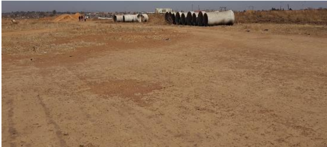
Fig. 62. Looking south from marker 6. Here the effects of ploughing, construction work and dumping can be observed. (Photo S.M. Miller 2020.)
