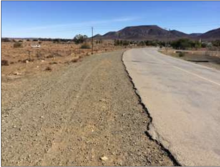
Figure 24. Proposed sewer route alongside R355 south
