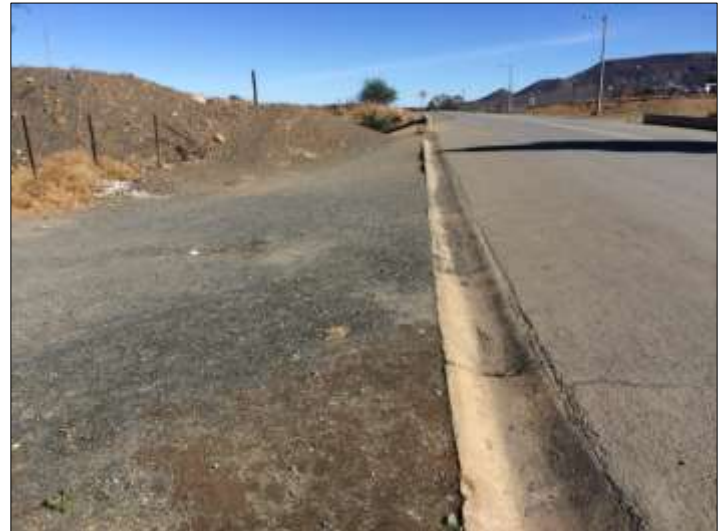
Figure 22. Proposed sewer route alongside R355 south
