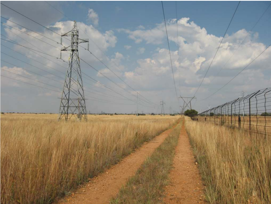
Photo 4: View of the power lines on the western side.
