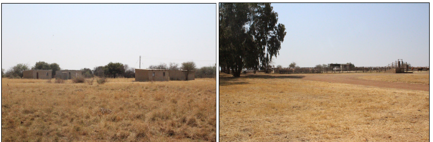
Figure 4.3: Farming infrastructure and workers houses identified on the Farm Zamenkomst No 04 Portion 02
