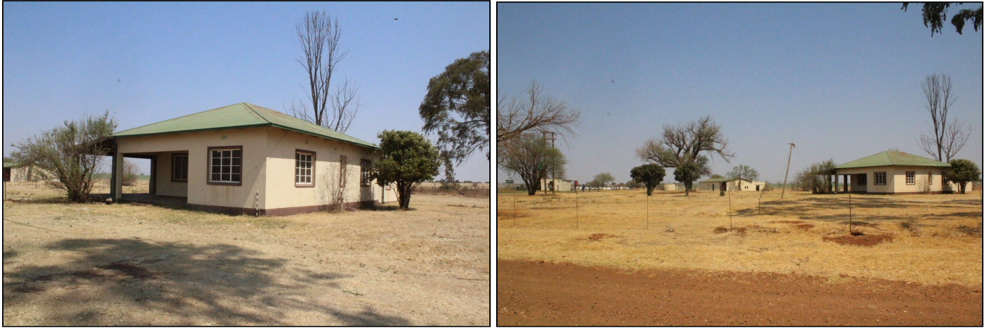
Figure 6.4 Southern Corner of the farm house and 6.5 Northern Corner of the farm house
