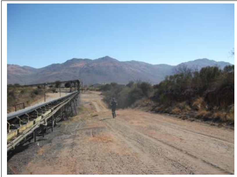
Figure 7- The existing Slag Overland Conveyer will be re-aligned from the Smelting Plant to the Slag Dump (above).
