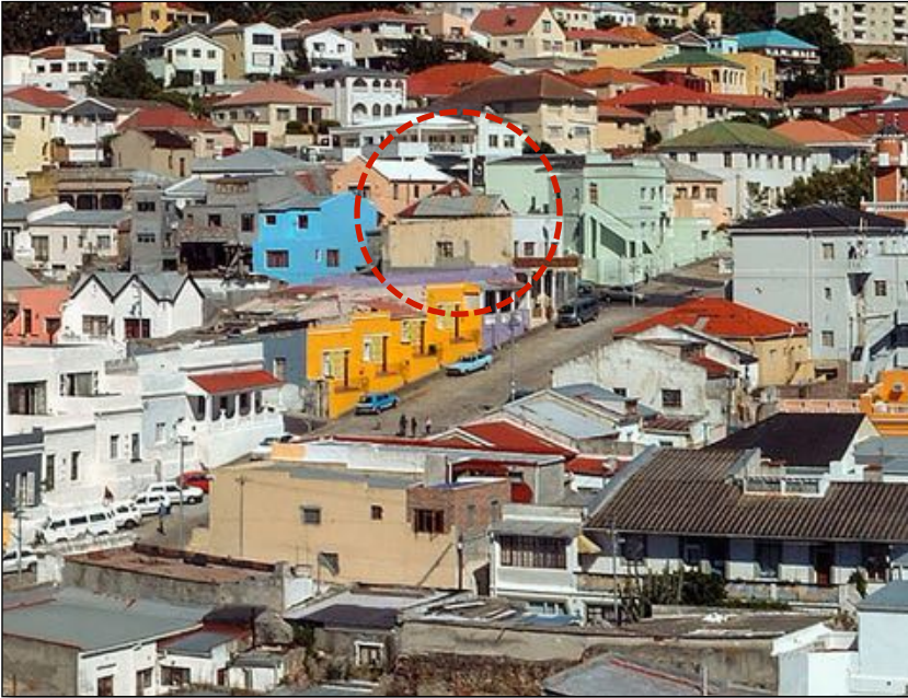
Figure 26: A view of Bo-Kaap, looking west, in 2001. The roof of 2 Lion Street (circled, then still intact, although showing signs of decay) can be seen protruding above the double-storeyed 67 Leeuwen Street (with red balcony). Leeuwen Street runs from bottom left to the top right. (Francois Swanepoel)
