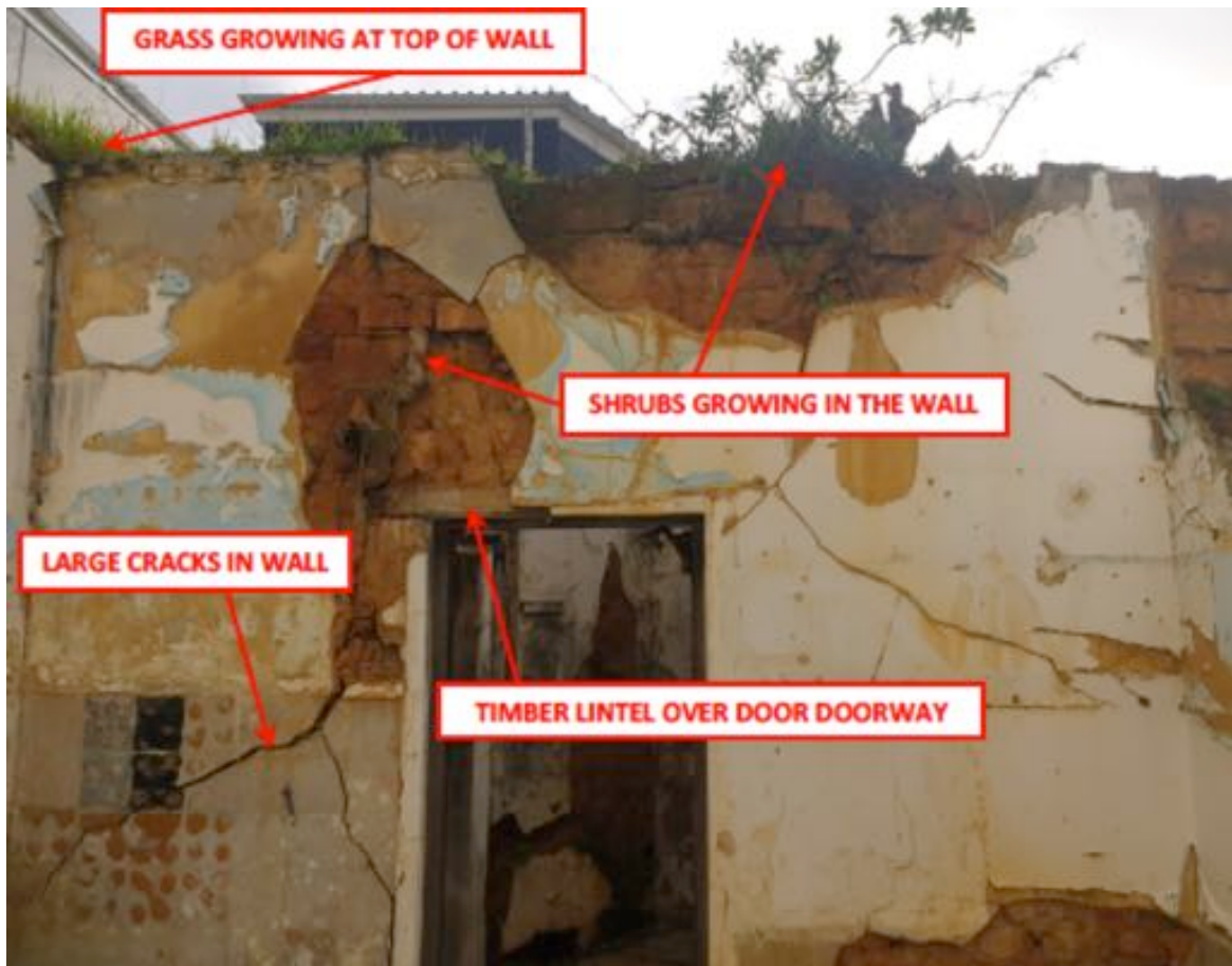
Figure 17: Waal panel with door opening (Abe-Struc 2020: 4)
