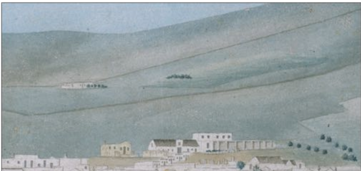
Figure 18: Part of the Josephus Jones c.1808 panorama, showing the flat-roofed Schotsche Kloof homestead (now 79 Dorp Street) at bottom centre, with its thatched and gabled outbuilding on its left. Leeuwen Street and Lion Street were later developed on what is seen here as open farmland behind the homestead. Schoone Kloof , another market garden homestead, is seen in the background. (Rembrandt van Rijn Art Foundation, Stellenbosch)
