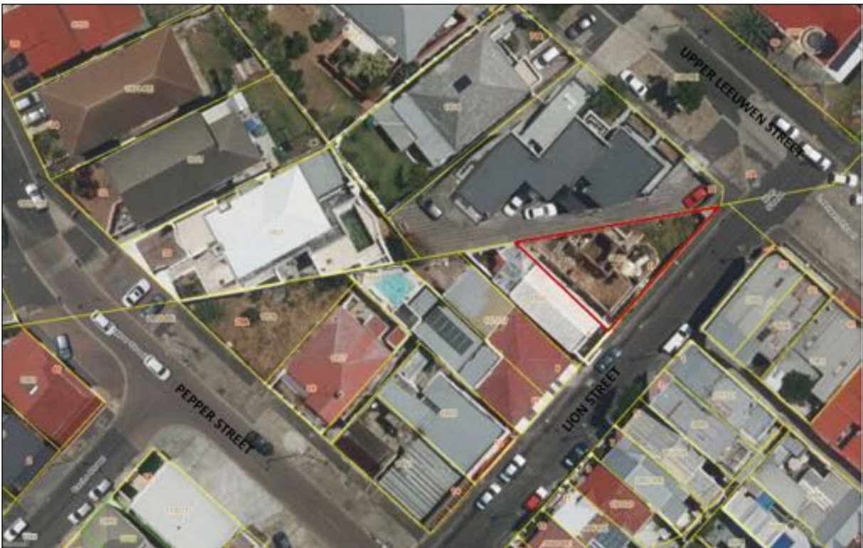
Figure 45: Detail of the government aerial survey of 2019. In the succeeding decade since the 2009 aerial survey (Figure 29), some of the inner walls of 2 Lion Street have collapsed. (CoCT Heritage Branch, Wale Street, Cape Town; annotated by J Hislop)
