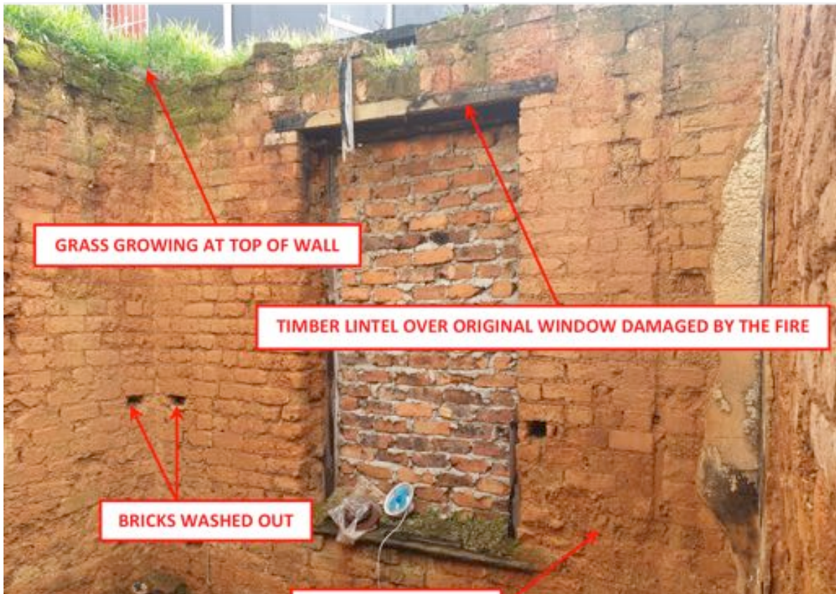
Figure 16: Original window construction (Abe-Struc 2020: 5)
