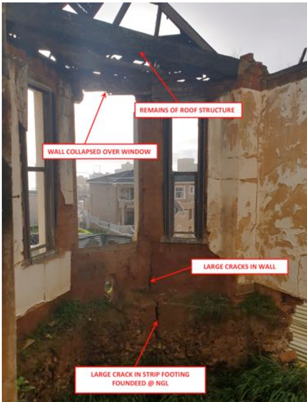
Figure 15: Bay window in lounge (Abe-Struc 2020: 6)
