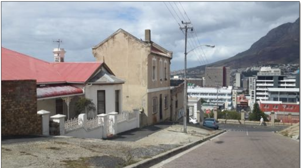
Figure 46: A view of Lion Street in the middle distance, as seen from Upper Pepper Street. The steep set of stairs (behind the stop sign) are a Lion Street landmark (built after c.1897; they are not shown on the Thom Survey, Figure 20), and lead down to the lower section of Pepper Street. The Victorian house on the left (Hillside Villa) is similar to the original building at 2 Lion Street, although the gable is more squat and it was designed by a different architect (W.T. Wilkinson, not Robert Esdon)(Hislop, 2016)
