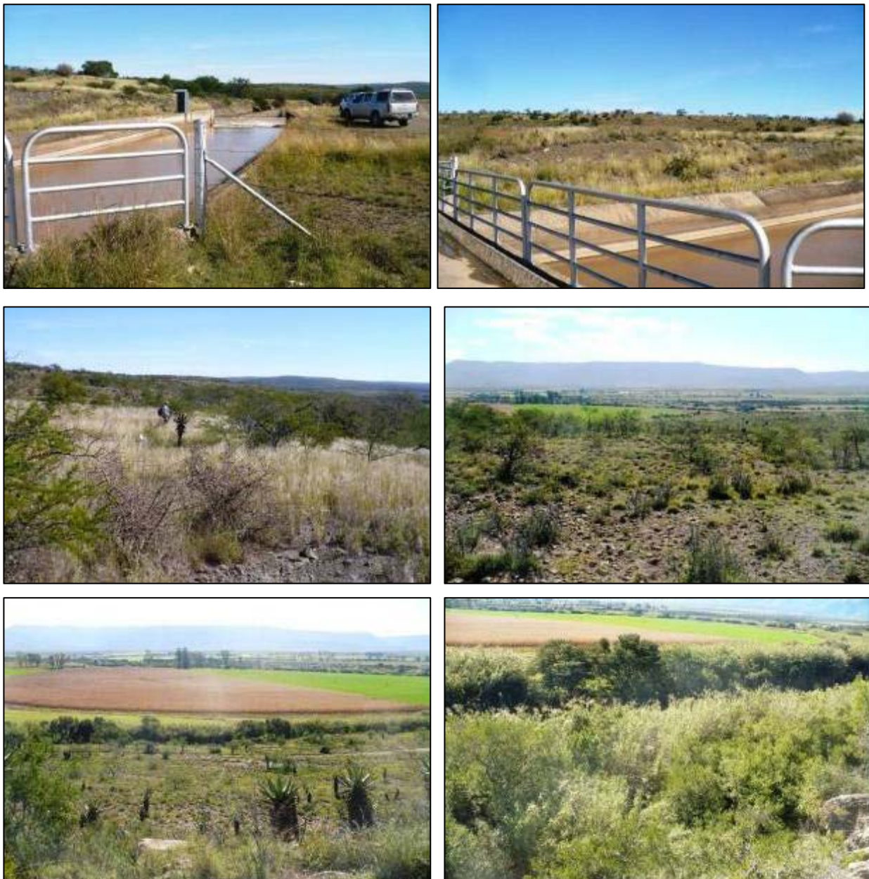
Figure 1. General views of the proposed site for the construction of the Little Fish Embedded Small Hydro.
