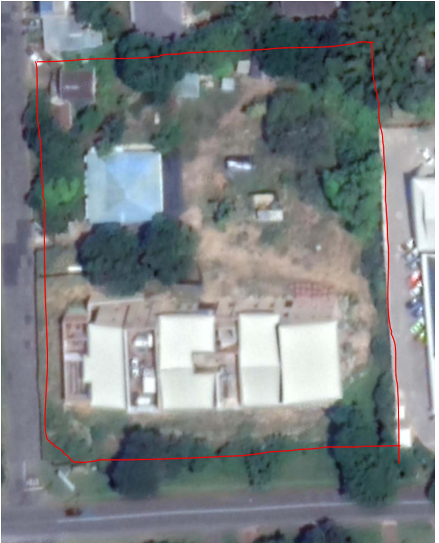
Aerial view of site:
