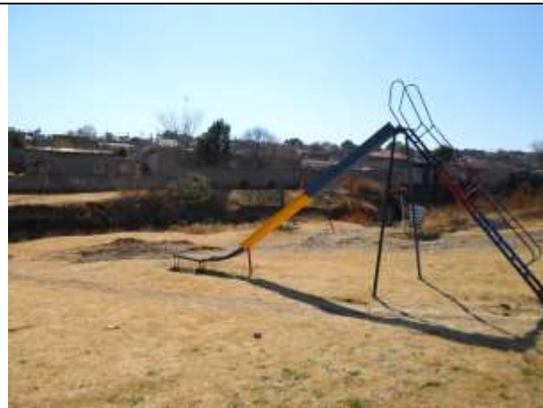
Figure 8. recreational park infrastructure.
